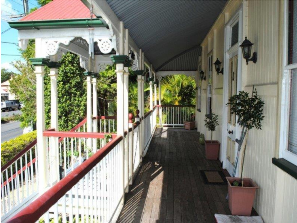
9 Warwick Rd, Ipswich, Front Veranda, detailing the VJ exterior walls and colonial style fretwork around the posts (Realestate.com, 2016c).
