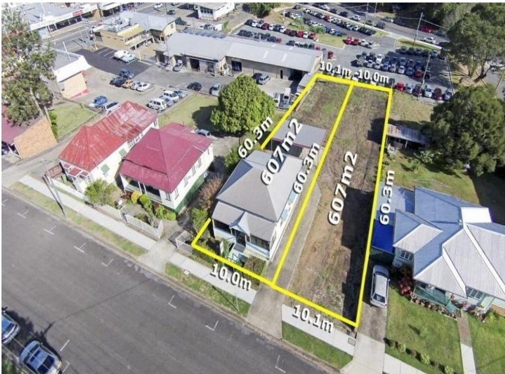
8 & 10 Mortimer Street, Aerial view(Realestate.com, 2016h).
