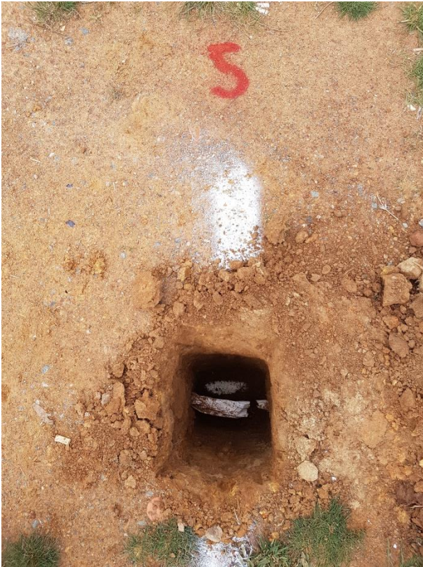
Figure 18. Photo at chainage 5 showing location of the underground utility line.
