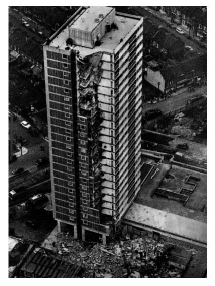
Figure 1-2. Gas explosion in the kitchen on the 18th floor of Ronan Point London 1968.
