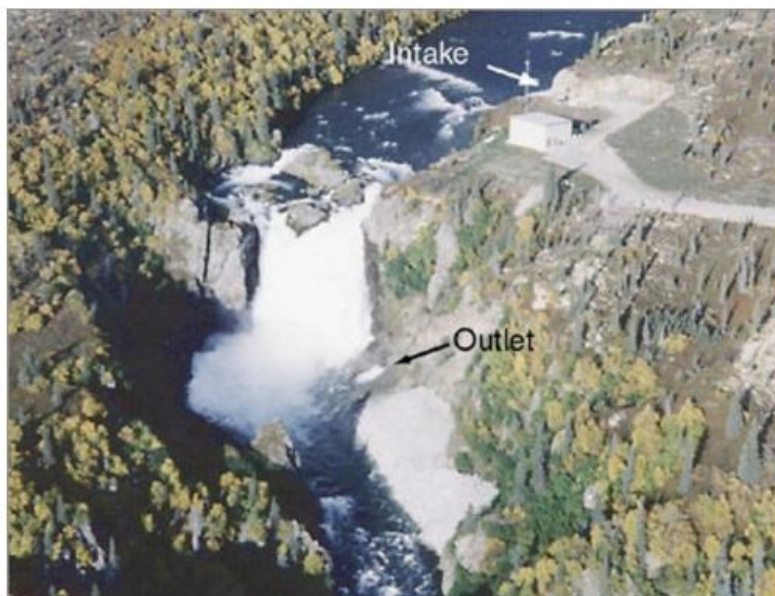
Figure 2.3; Diversion system in place (U.S. Department of Energy , 2013)
