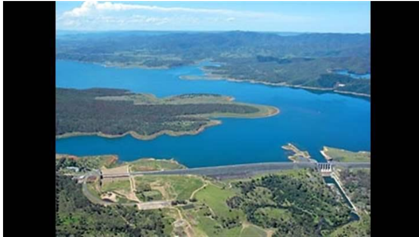
Figure 5.1: Aerial photograph of existing infrastructure
