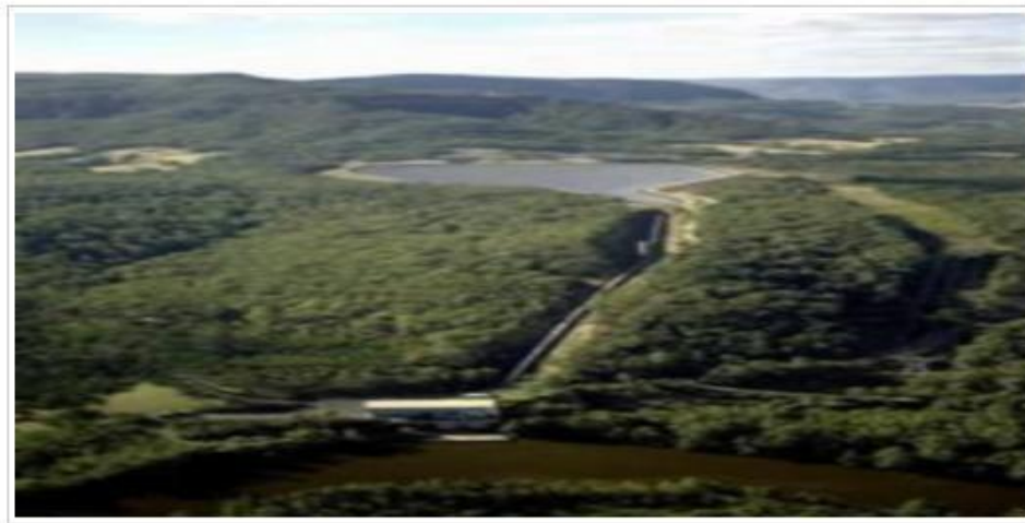
Shoalhaven, Eraring Energy
