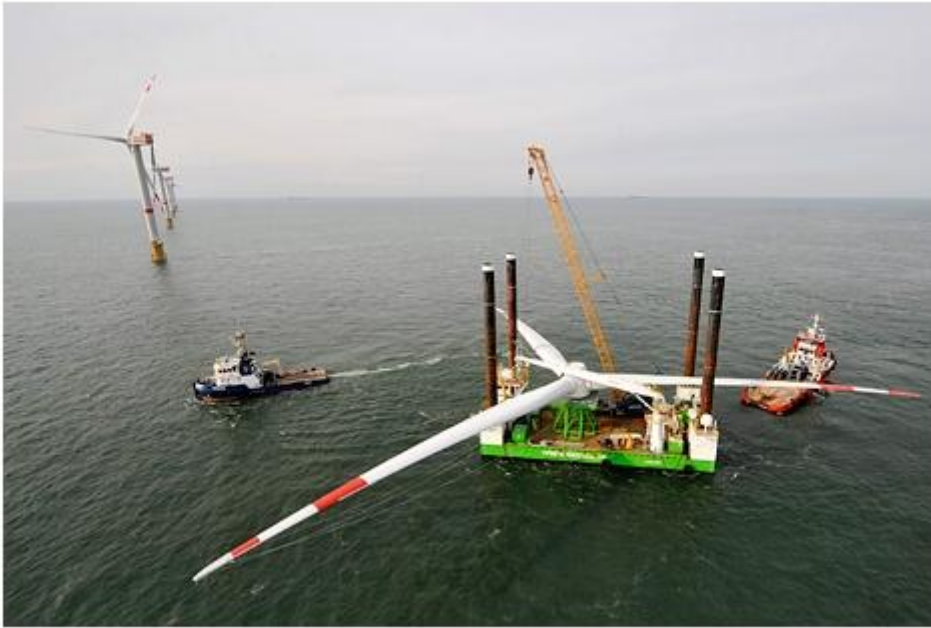
Figure 2.27; Offshore wind turbine construction
