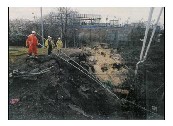
Figure 5.4: Sinkhole caused by blowout (Institution of Civil Engineers 1998).
