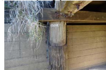
(b) Vertical splitting (pile)
