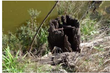
(a) Splitting (girder with a fastener)
