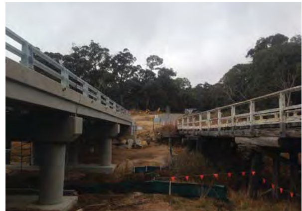
Figure 1 - New and old bridges
