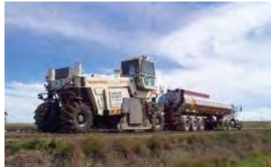
Figure 1: In situ foamed bitumen stabilisation (Kendall, Baker, Evans, & Ramanujam, 2016)
