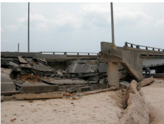
Figure2-7: Damage caused by scouring (Padgett et al. 2008)
