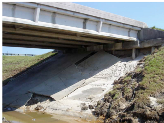
Figure2-7: Damage caused by scouring (Padgett et al. 2008)
