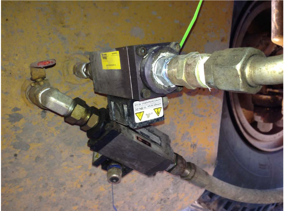
Figure 15: Installation of Kral Volumeters to fuel tank of Caterpillar 785D truck (Kubler 2015)
