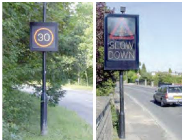
Figure 4.7: Speed-activated speed limit sign
