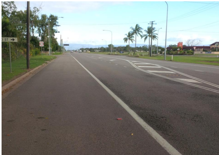
Figure 6.16: Ingham south approach (facing south)
