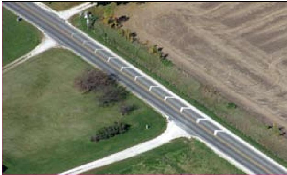
Figure 4.18: Converging Chevrons installed at Roland, USA
