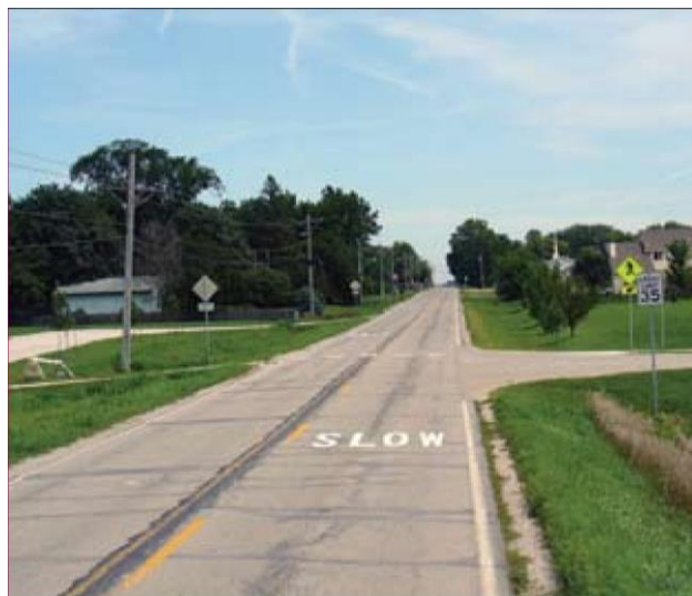
Figure 4.20: “SLOW” pavement legend in Slater, USA
