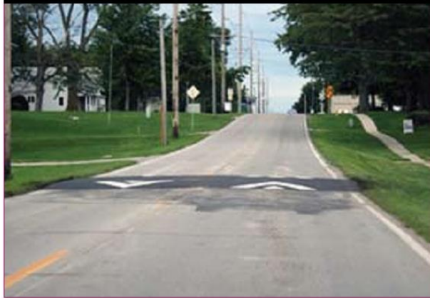
Figure 4.22: Driver view of speed table in Gilbert, USA
