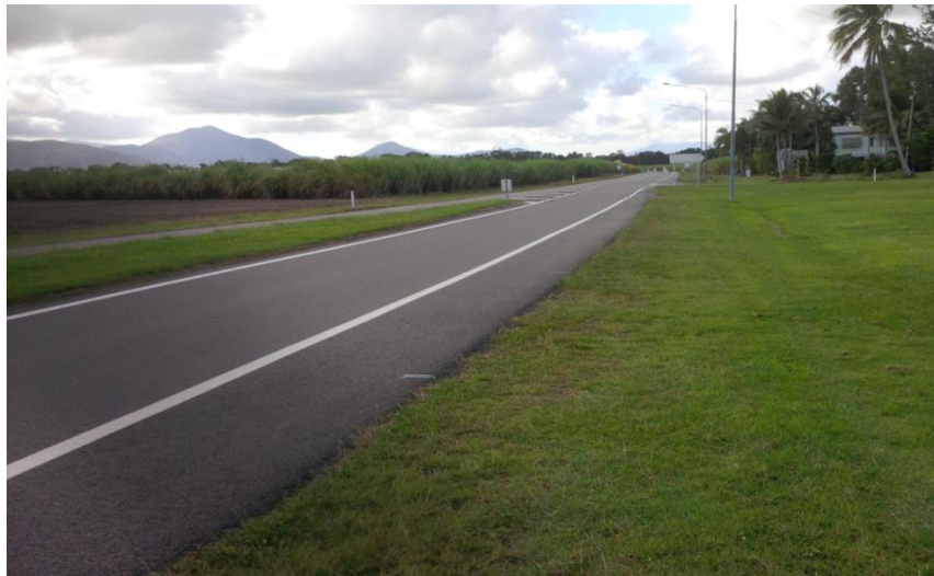
Figure 6.10: Ingham north approach (facing north)
