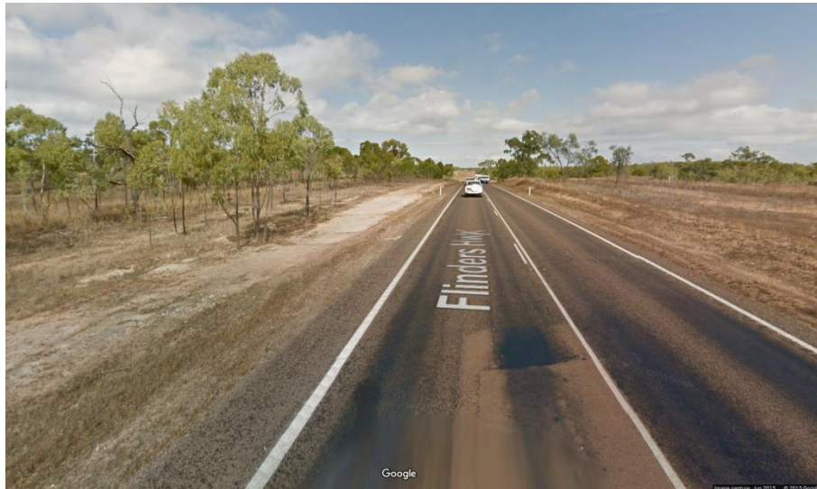
Figure 1.3: Typical depiction of Flinders Highway (Townsville to Charters Towers)
