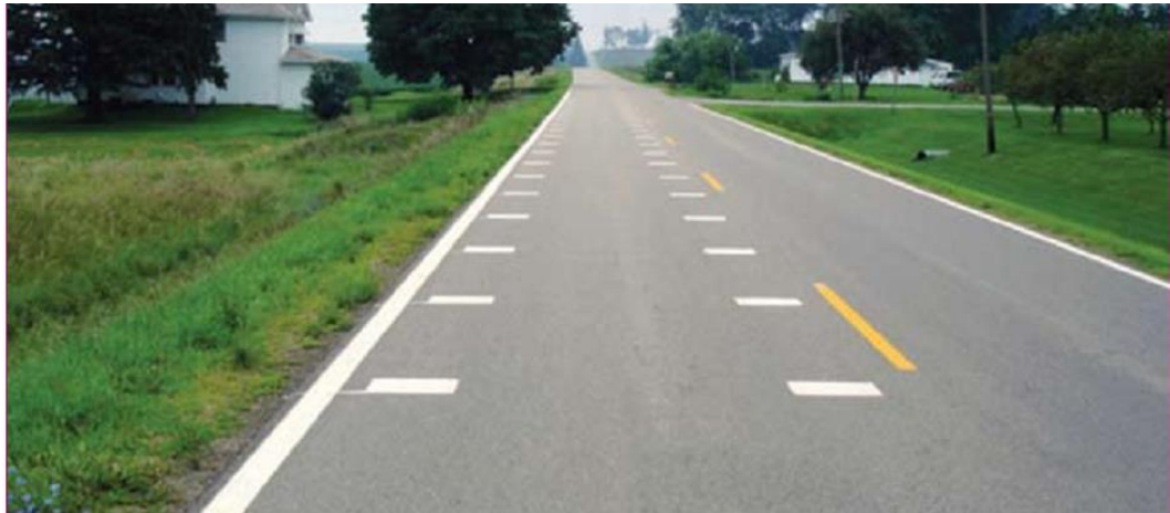
Figure 4.12: Experimental transverse markings at entrance to Union, USA
