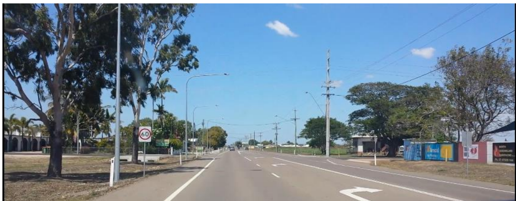
Figure 6.29: Ayr north approach (facing south)
