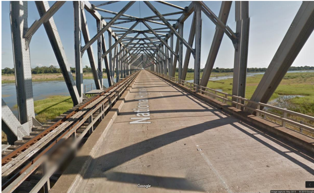
Figure 3.4: Burdekin Bridge facing north
