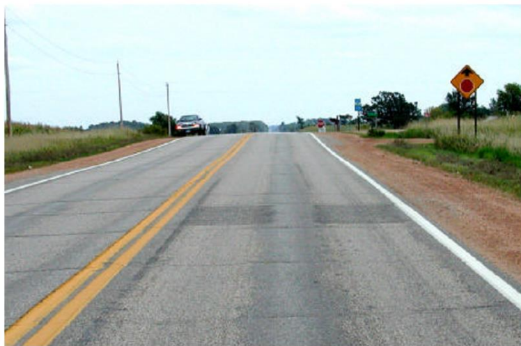
Figure 4.9: Rumble strip – wheel paths only
