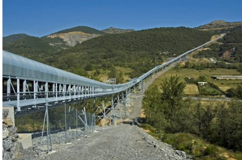
Figure 2.3: Troughed belt conveyor (BEUMER 2012)
