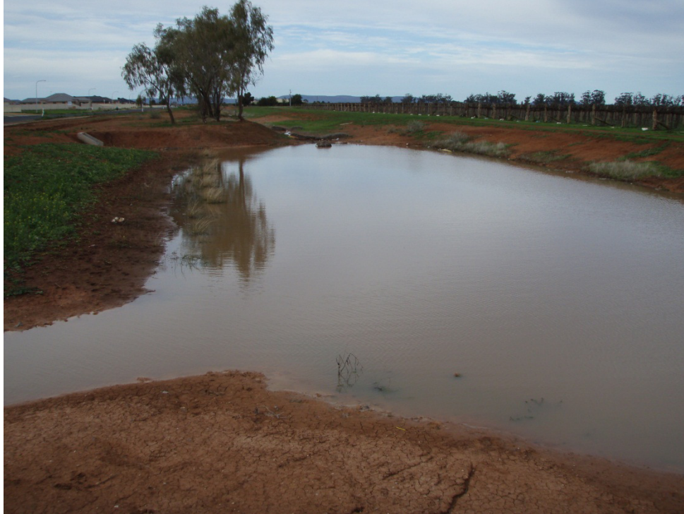
Figure 8 – Study Area Drainage Channel retention system, where a 100 residential lot development discharges stormwater runoff.
