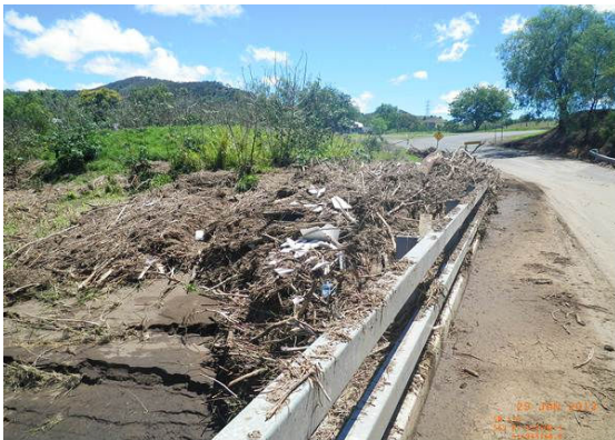
Figure 1: Damaged Bridges in Lockyer Valley Region in Queensland
