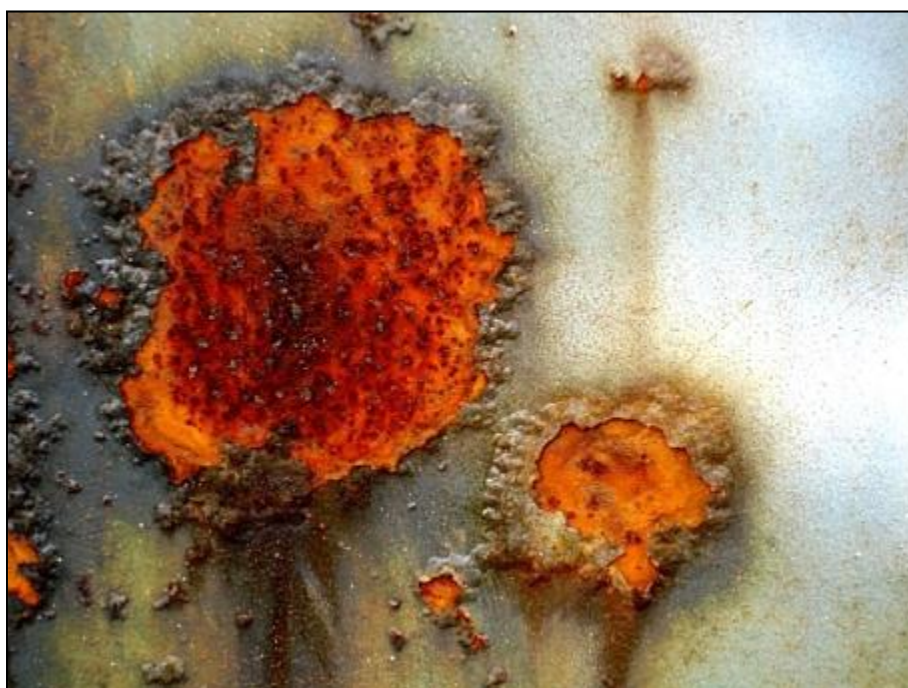
Figure 1.2 Corrosion on steel surface in saline environment (Green Cleaning Ideas 2011)
