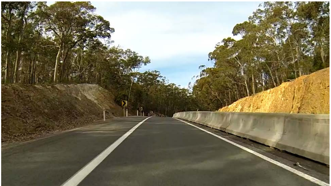
Figure 11 – Horizontal curve concealed by sharp vertical crest on southbound carriageway, Princes Highway, Dalmeny.
