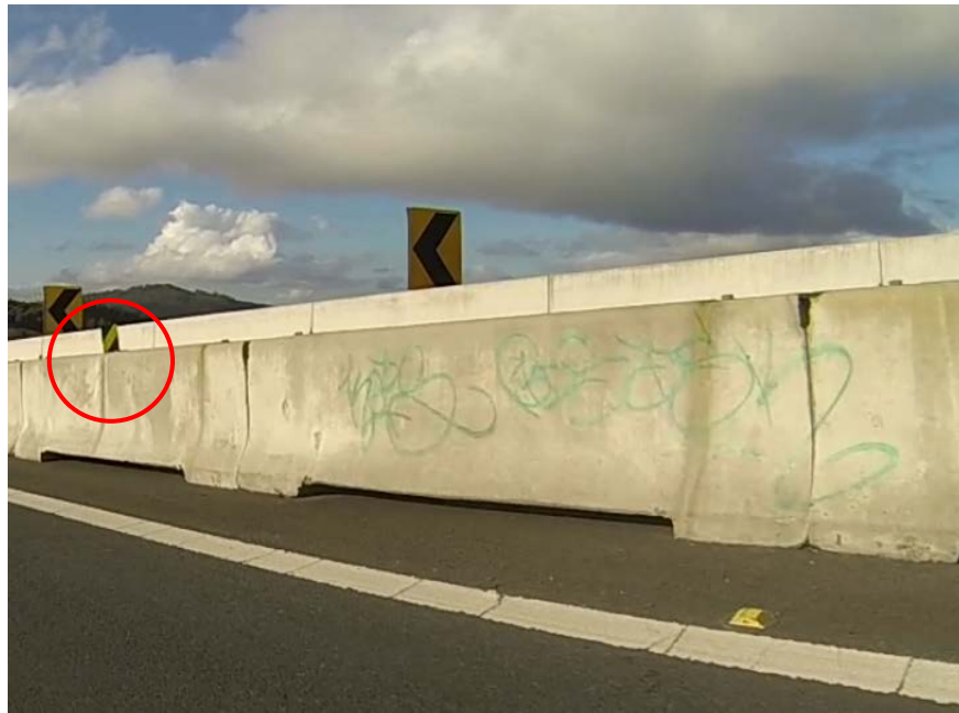
Figure 19 – Robertson graffiti and metal curve alignment markings fixed to the central barrier (red)
