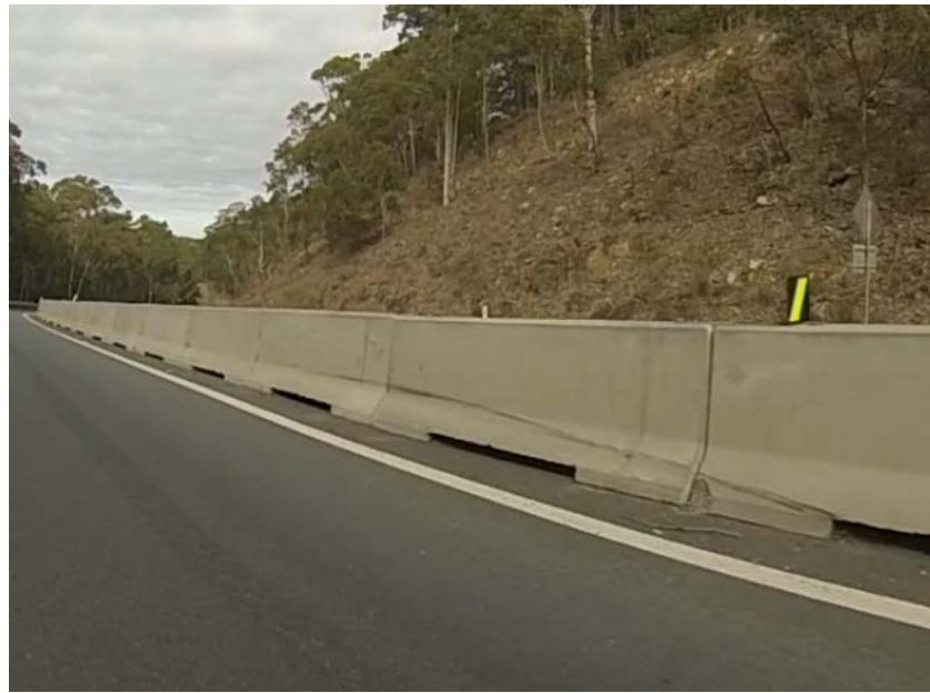
Figure 13 – Batemans Bay central safety barrier ramping
