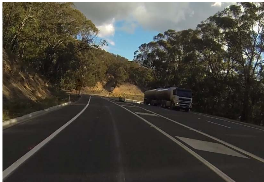
Figure 22 – Mount Victoria Pass (bottom) removed chevron, westbound approach
