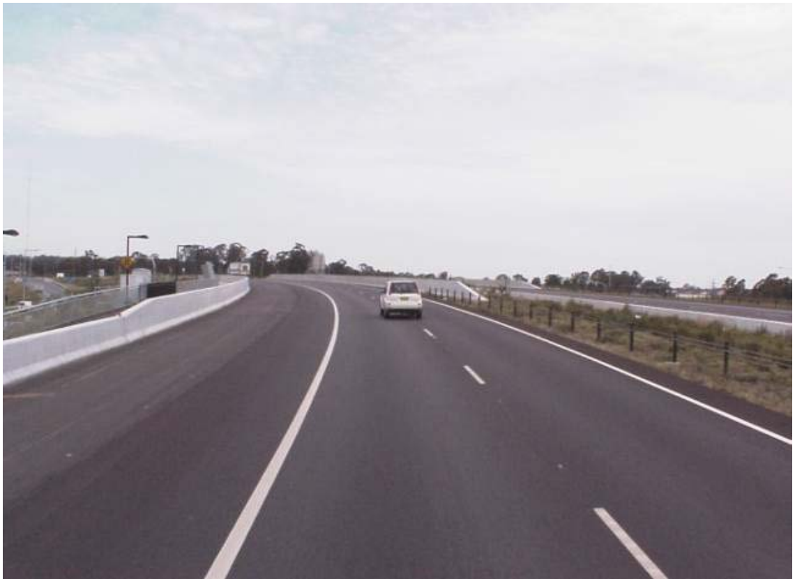
Figure 8 – SD widening on the Sydney Ring Road (Arndt et al, 2009)
