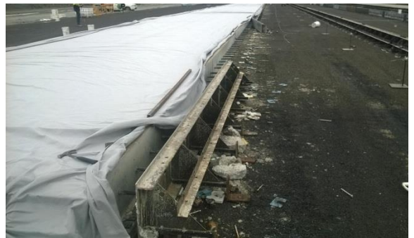
Step 10- Removal of formwork 1 day after paving
