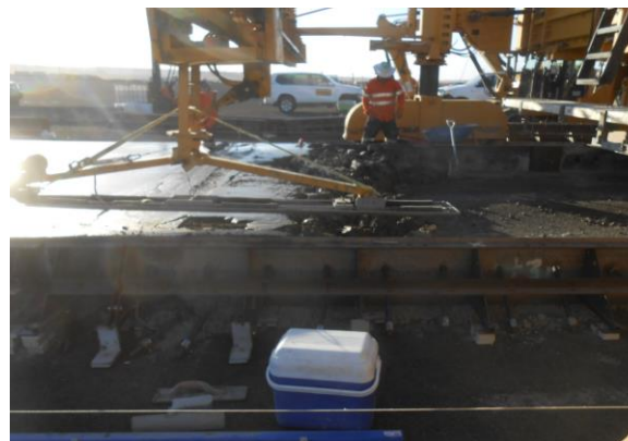
Step 4 – Paver moving over skipped bay
