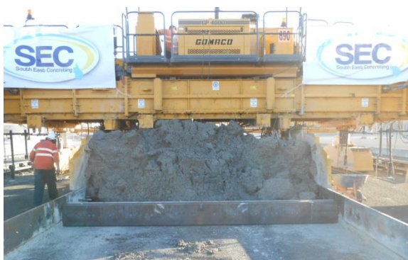
Step 3– Installed formwork which paver can move over
