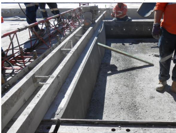
Step 3 - Placement of foam expansion joint.
