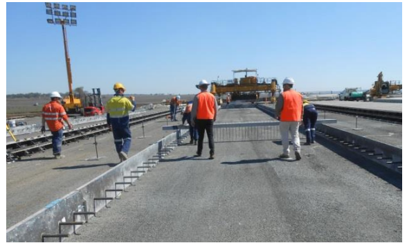
Step 8 – Scratch test to check formwork height
