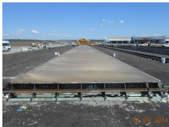
Step 9 – Completed concrete run.
