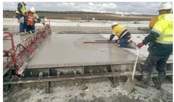
Step 8 – Screeding surface
