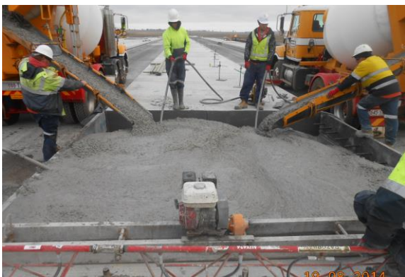
Step 6 – Pouring bay using chutes on two concrete trucks.
