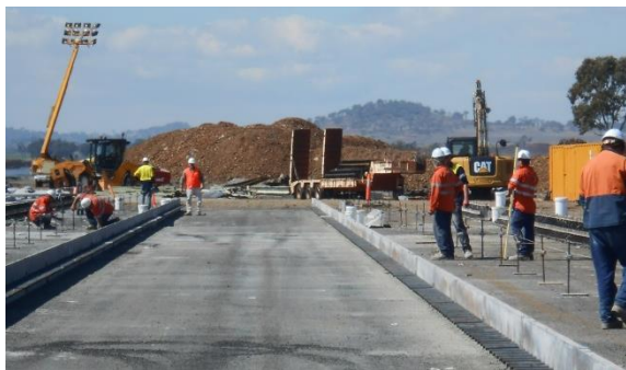
Step 9 – Finished formwork run ready for paving
