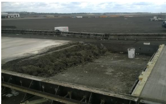
Step 1- Hand pour bay after paver has passed
