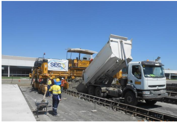
Photo 3 – Placement of concrete in front of terminal.
