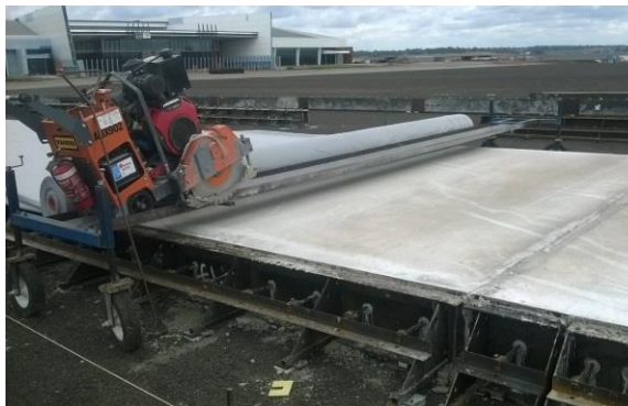
Photo 5 – Softcut surface to induce cracking. And placement of geofabric to slow curing.
