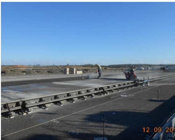
Step 11 – Cleaning out sawcuts .
