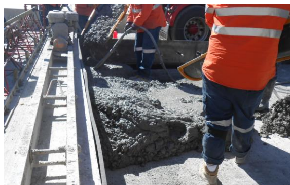
Step 6 – Pouring bay using chutes on two concrete trucks.
