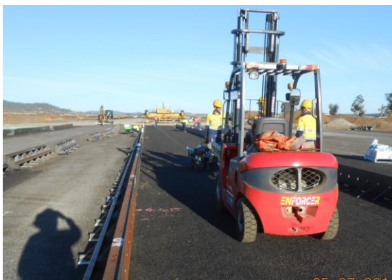
Step 3– Moving generator for drill along run.
