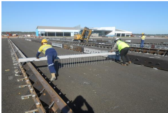
Step 1 - Conducting scratch test before concreting can commence.
