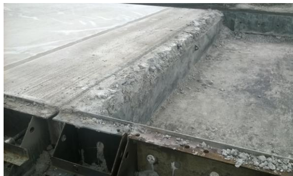
Step 2 – Cleaned face of slab for installation of expansion joint
