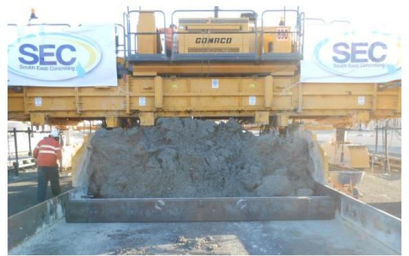
Photo 4 – Installation of the end-of-run formwork.
