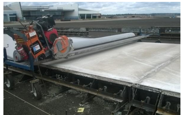
Step 10 – Softcutting concrete surface to induce cracking.
