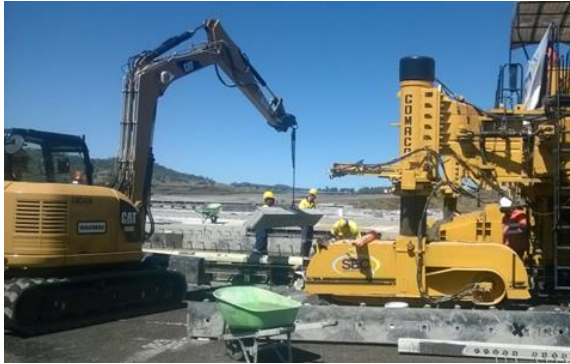
Photo 1 - Placing formwork for an expansion joint.
