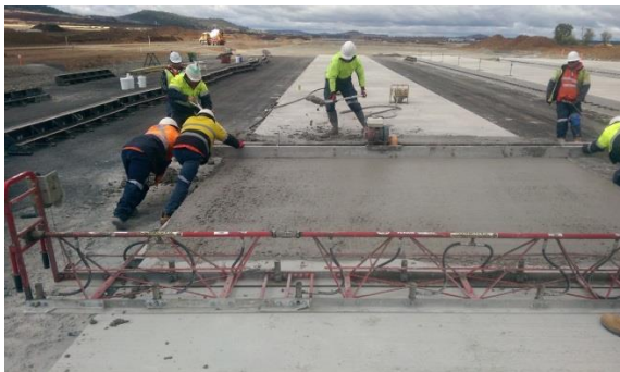
Step 7 – Placing concrete using a vibrating screed.
