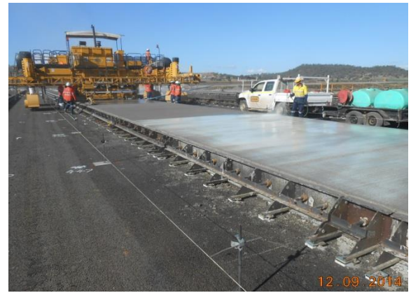
Step 8 – Concrete sprayed with curing compounds.
