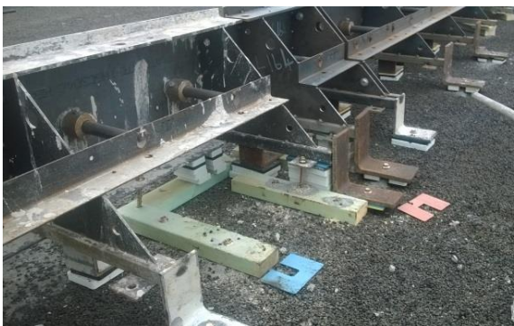
Step 5– Packers installed to height and forms bolted down on top
