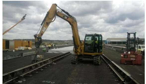
Step 2– Excavator lifting forms into place.
