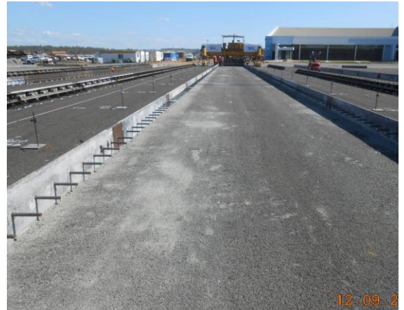
Step 2 – Setting up paver for run.
