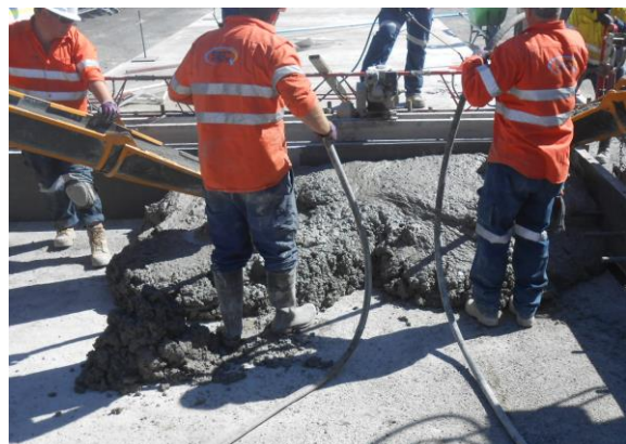
Step 5 – Vibrating concrete into place.
