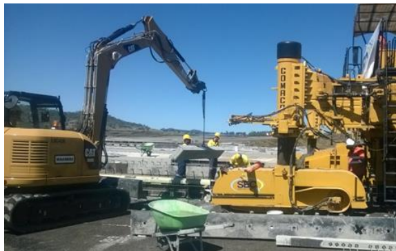
Step 3– Installed formwork which paver can move over
