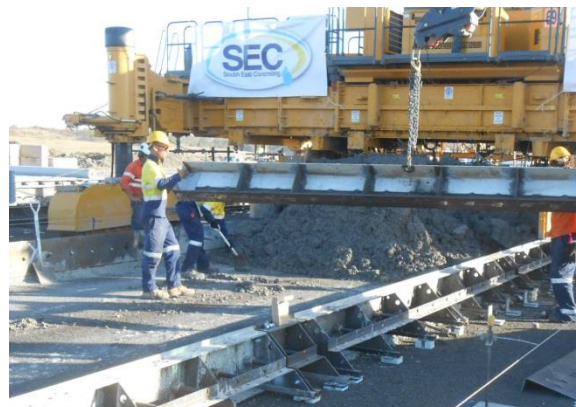
Step 4 – Paver moving over skipped bay
