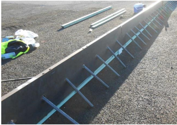
Step7- Dowel bars inserted into formwork
