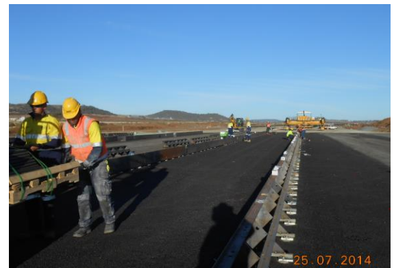
Step 4– Transporting dowels down run using forklift.
