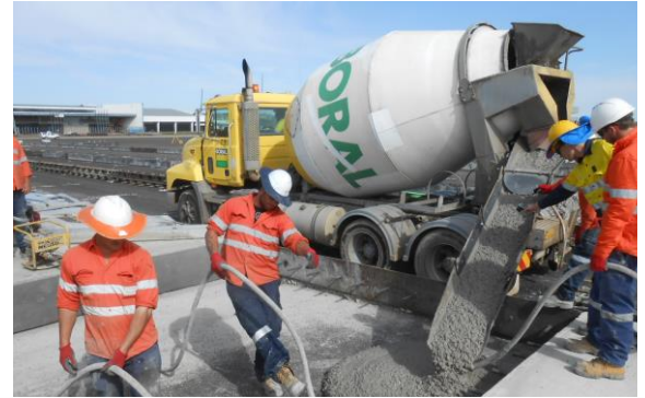
Photo 2 - Outsourcing concrete cartage to Boral for hand-pours.
