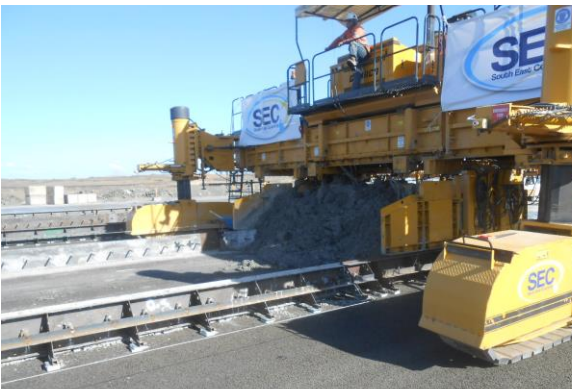
Step 5 – Paver pushes concrete forward vibrating the concrete into place.
