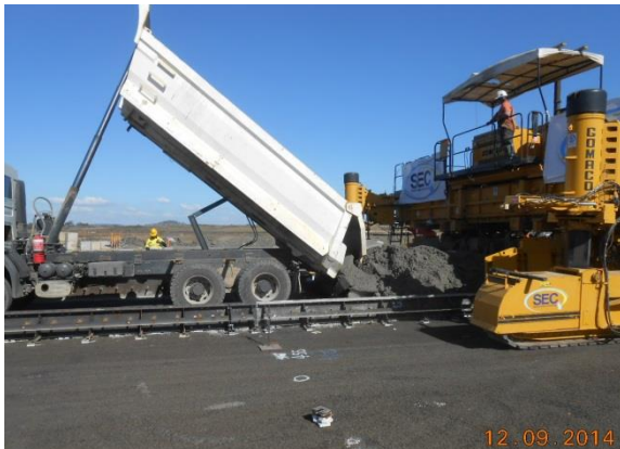
Step 3 – Dump truck tipping concrete in front of paver
