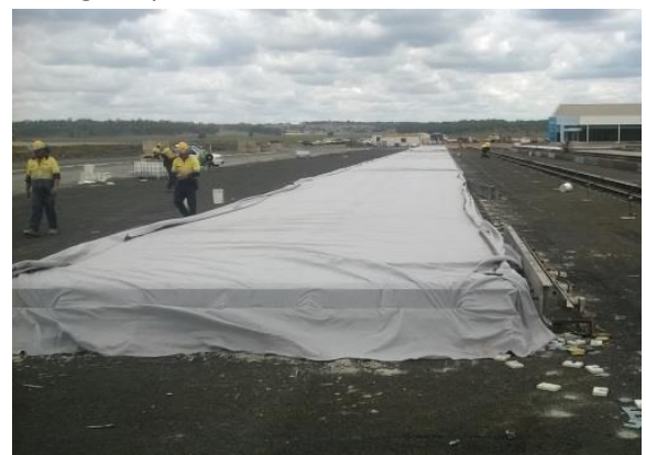
Step 12 – Covering with geofabric to enable curing in optimum conditions.
