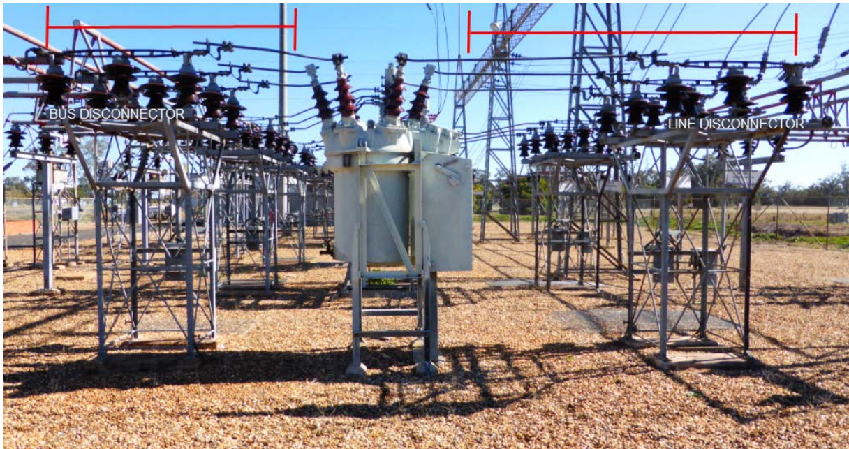
Figure 33: Circuit breaker 12 Section Safety Clearance.
