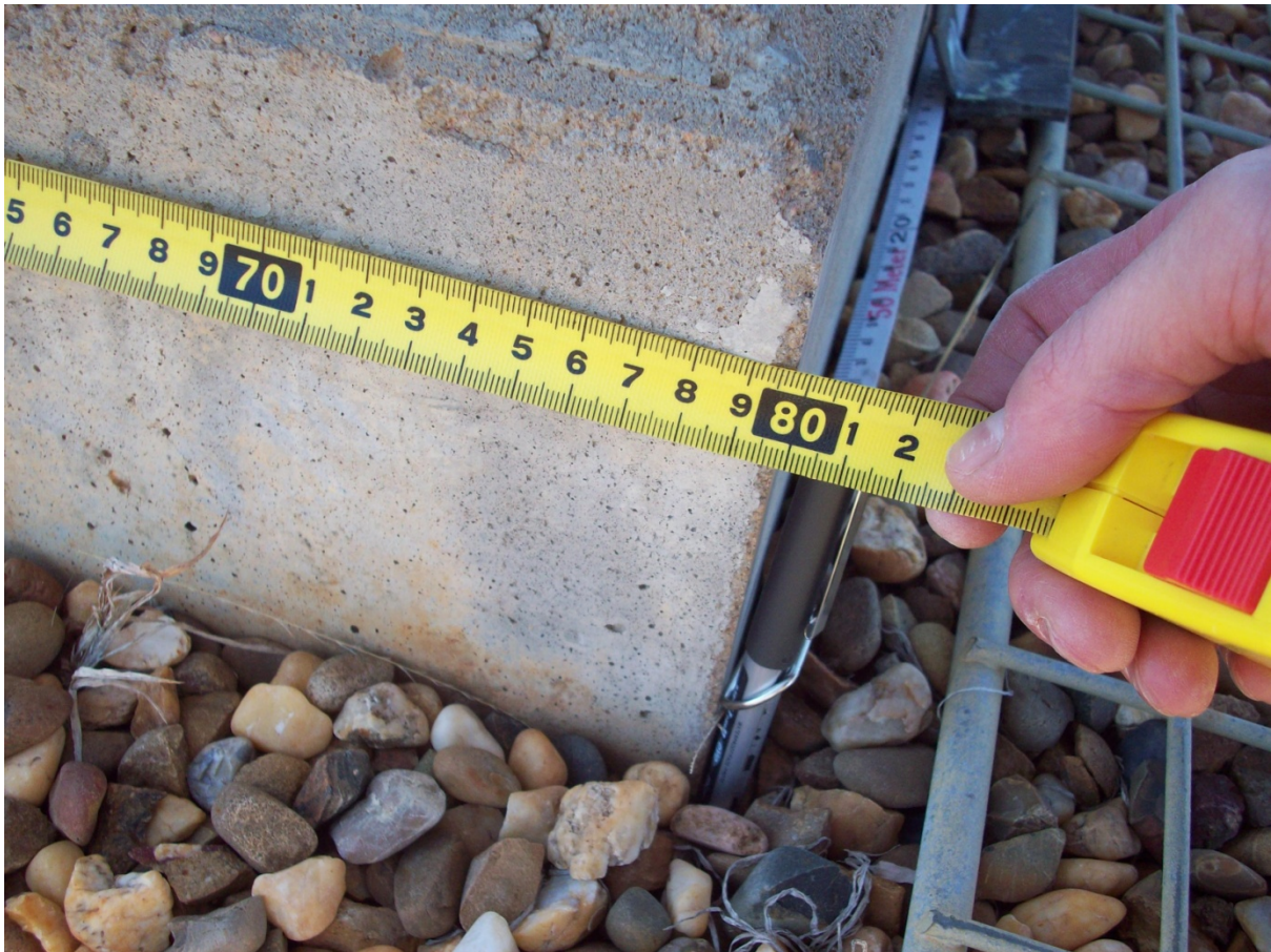
Figure 20: Item 1 132kV disconnecter, left concrete pad left side measurement.
