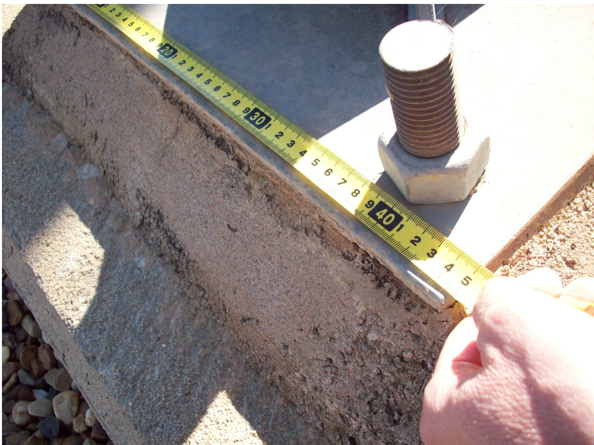
Figure 21: Item 4 132kV busbar support, right steel base plate rear measurement.
