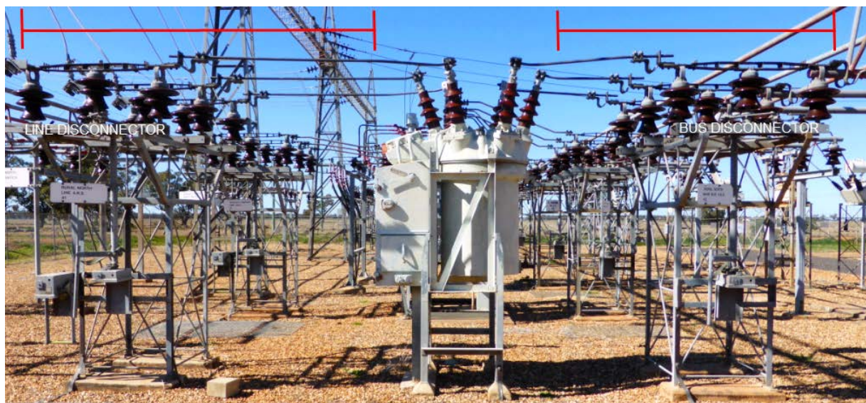
Figure 51: Circuit breaker 42 section safety clearance.
