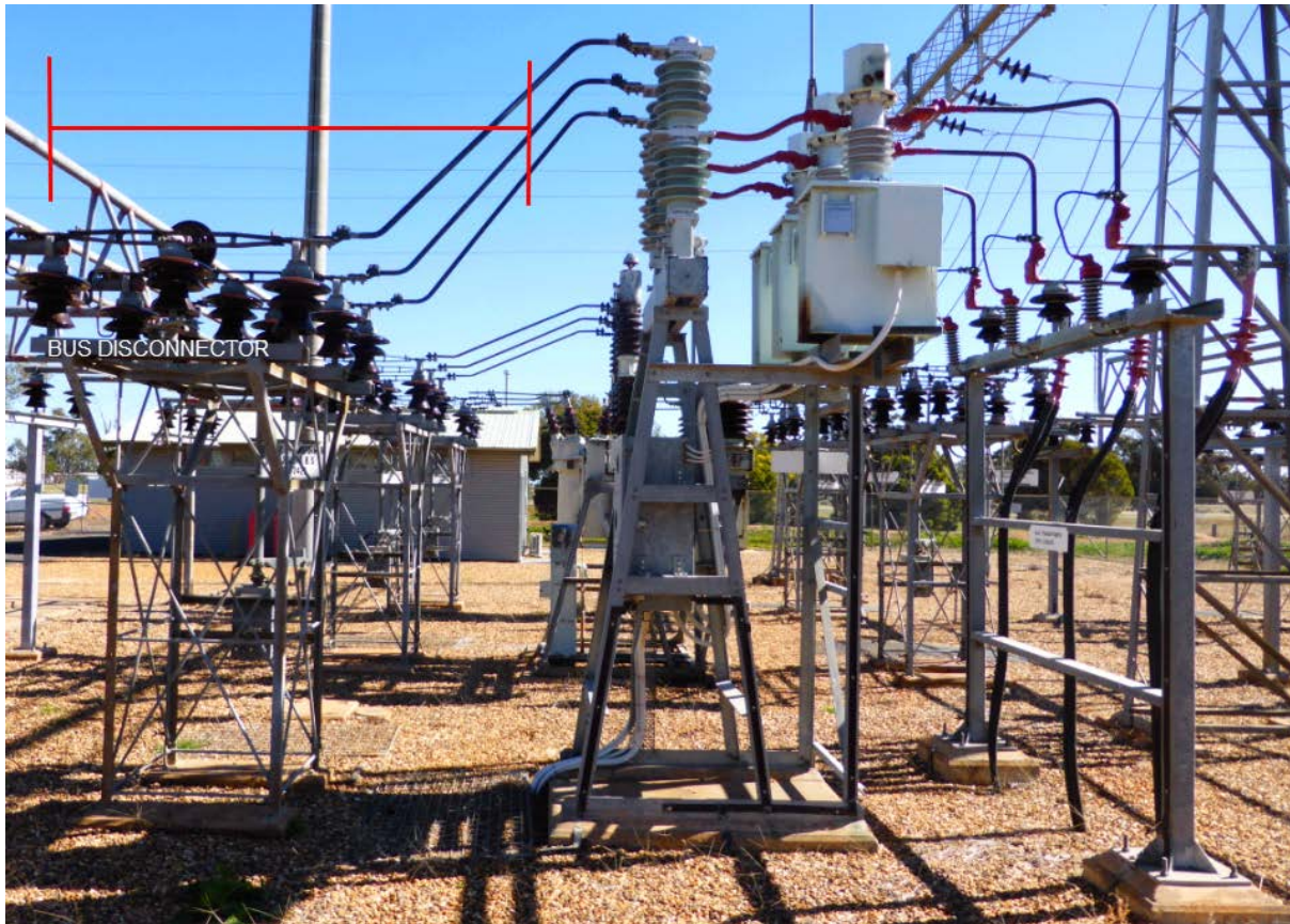
Figure 44: Transformer circuit breaker 2422 section safety clearance.
