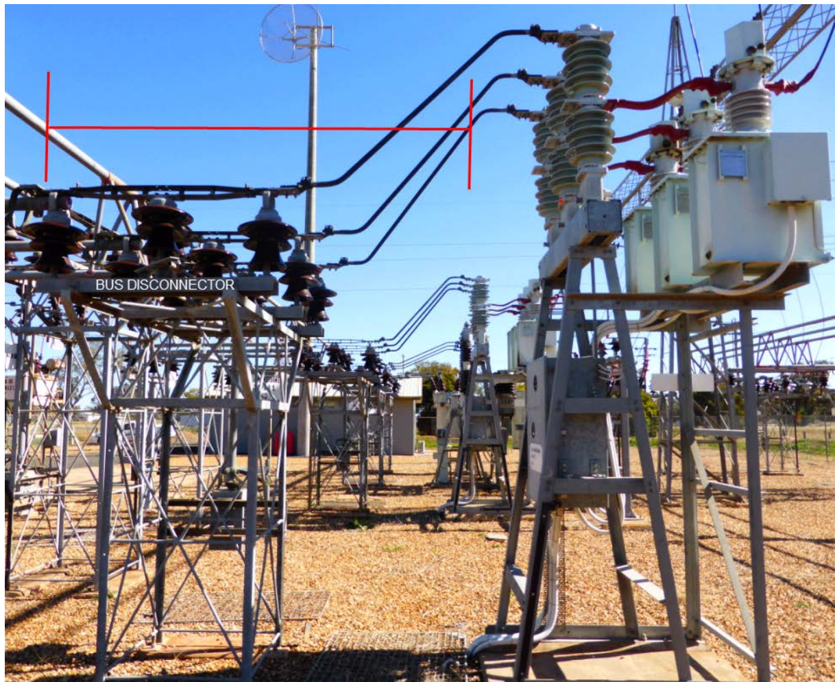
Figure 41: Transformer 2412 section safety clearance.
