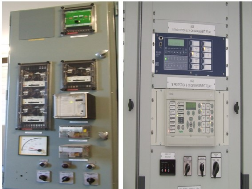
Figure 7-1 – Typical Protection Panel – Existing vs Test Facility
