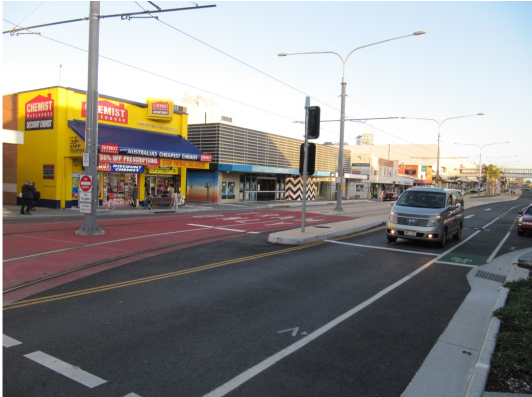
Figure 4.43 – Photograph showing the separation of tram tracks, vehicle lanes and bike lanes
