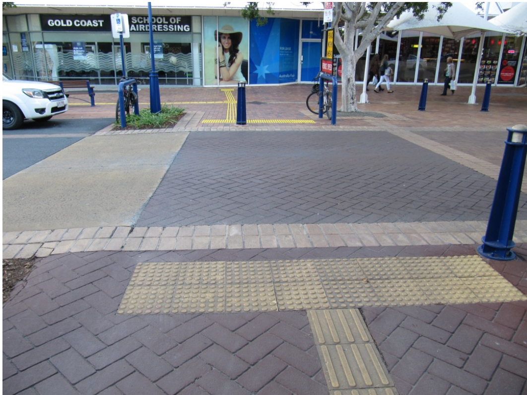
Figure 4.31 – Low speed road pedestrian crossing with tactile surface
