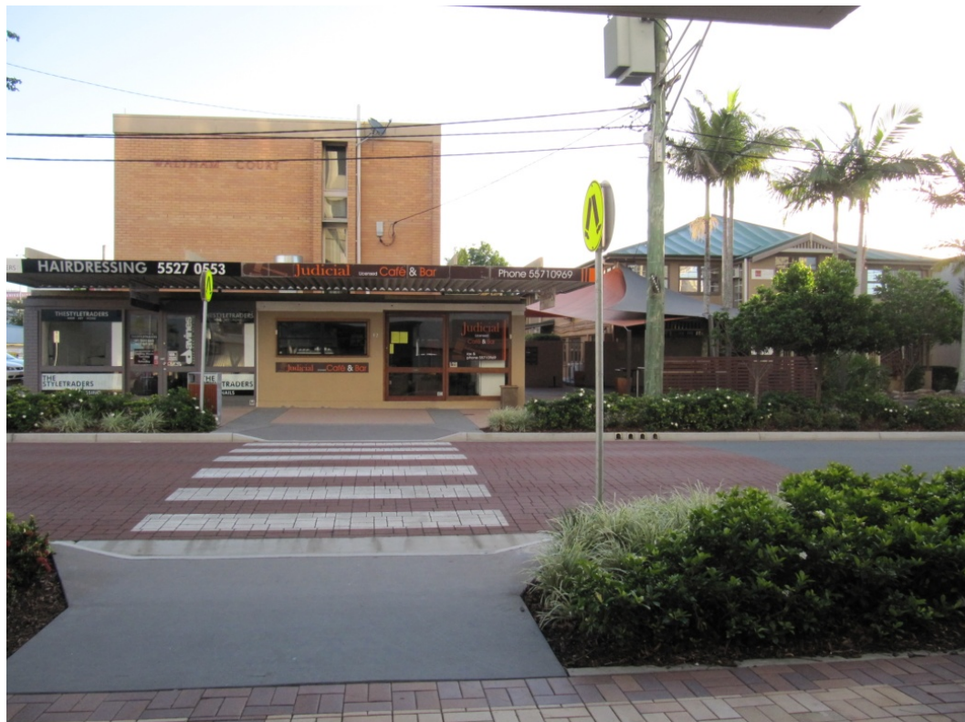
Figure 4.22 – Example of cafes and businesses along the route with residential units above
