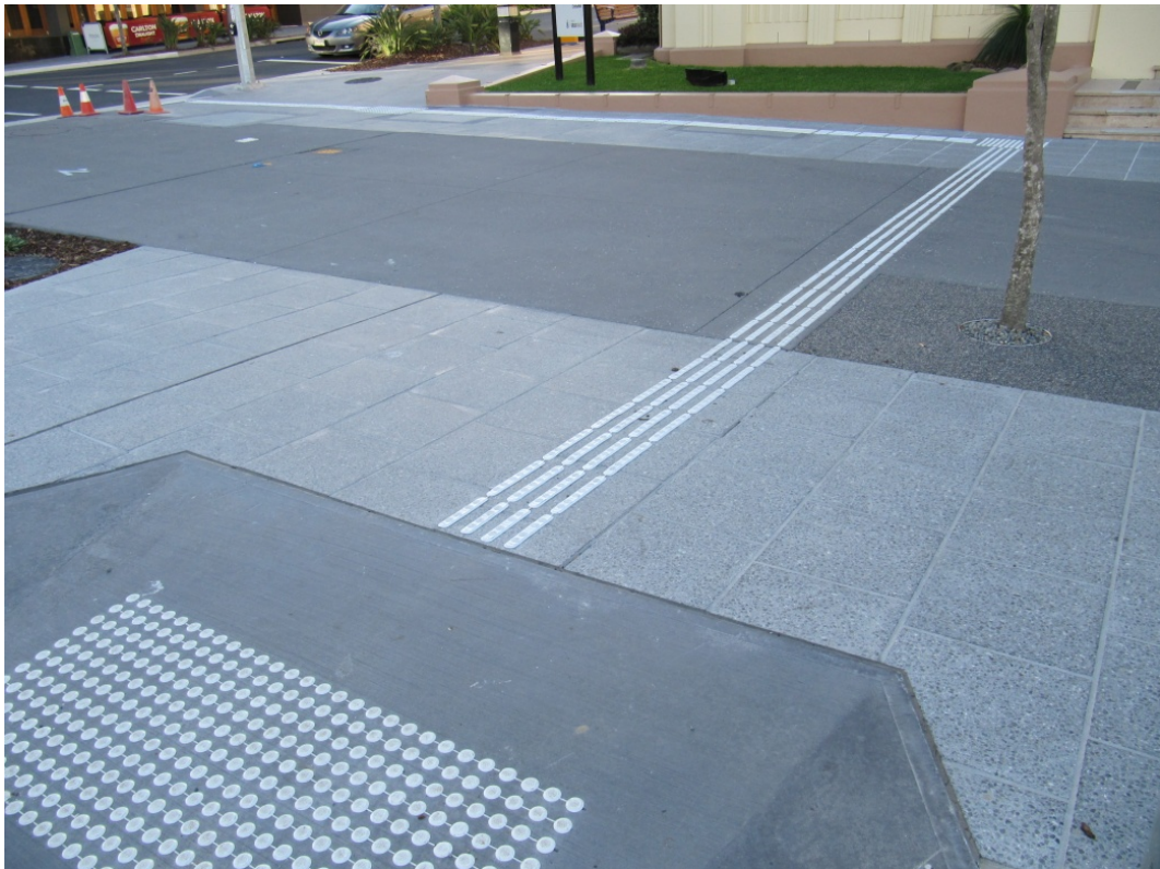
Figure 4.5 – Tactile surface for vision impaired pedestrians
