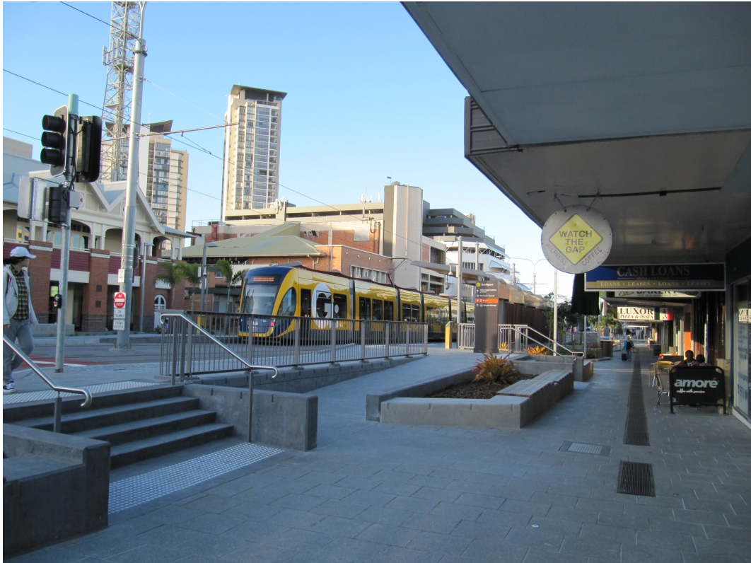
Figure 4.4 – Steps and ramps for access to the station platform
