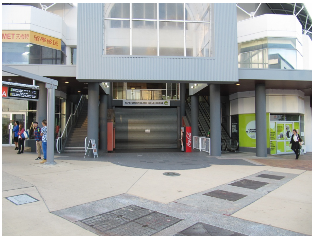
Figure 4.24(a) – TAFE and bus stop in front
