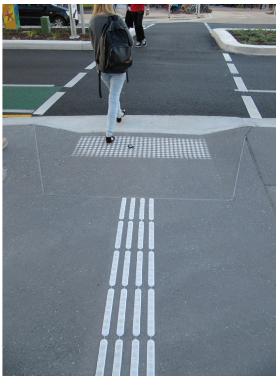
Figure 4.25 - Tactile surface and adequate waiting area at the crossing
