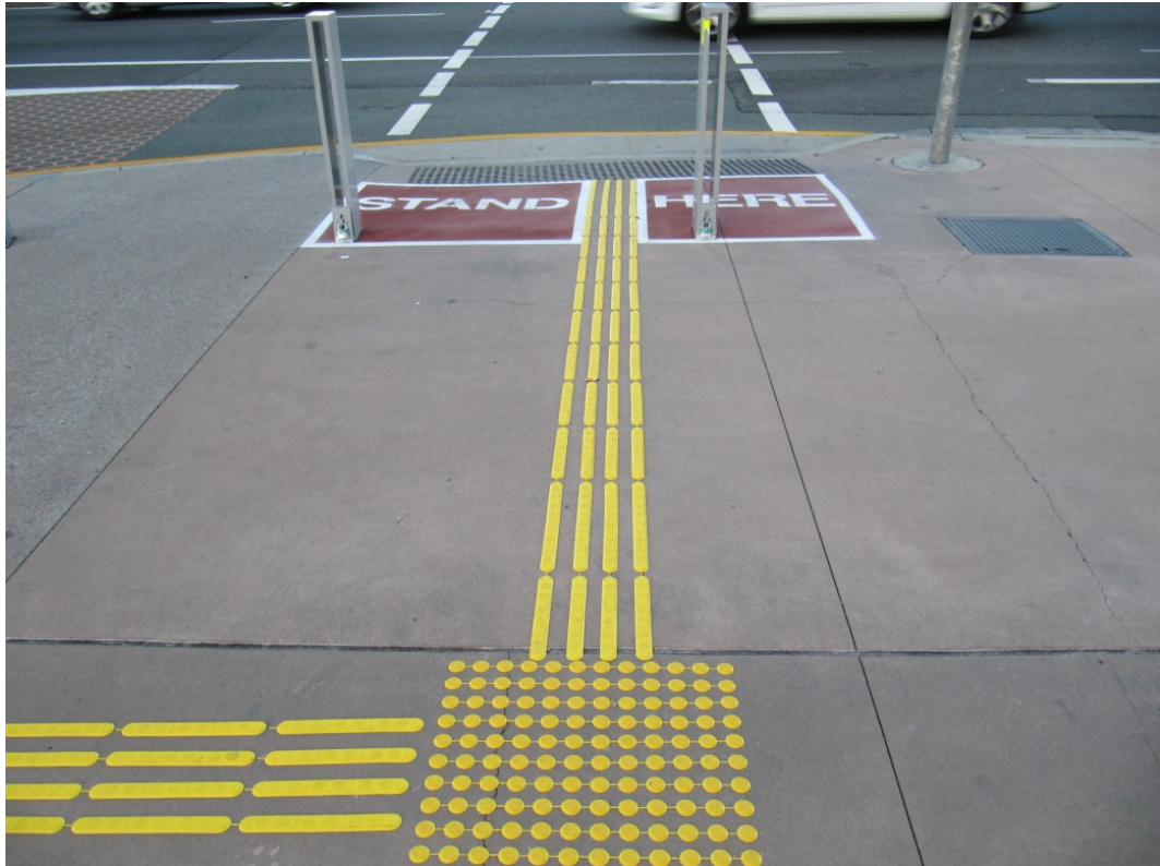
Figure 4.32 – Kerb ramp, safety bollards and tactile surfaces at the crossing of the Gold Coast Highway
