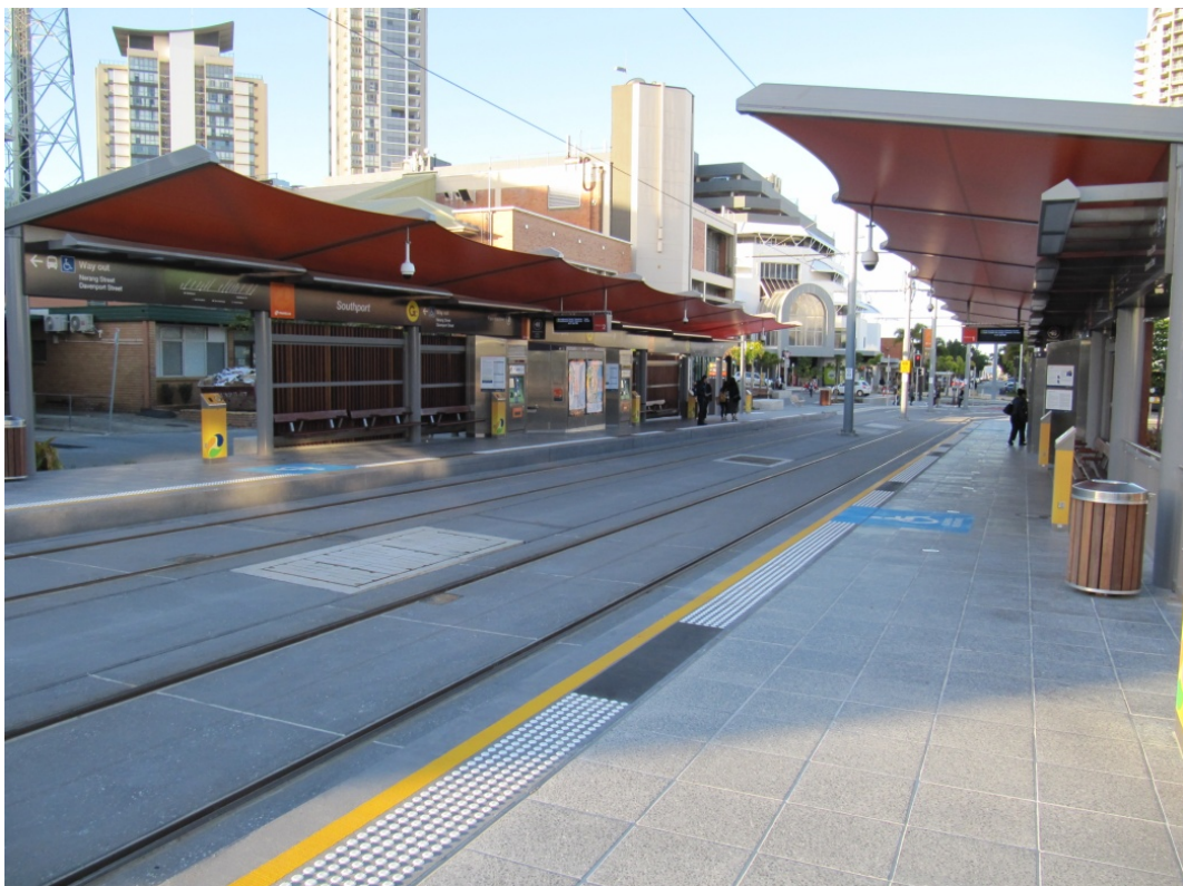
Figure 4.8 – Looking east on Station 5 platform with benches, seats and rubbish bins
