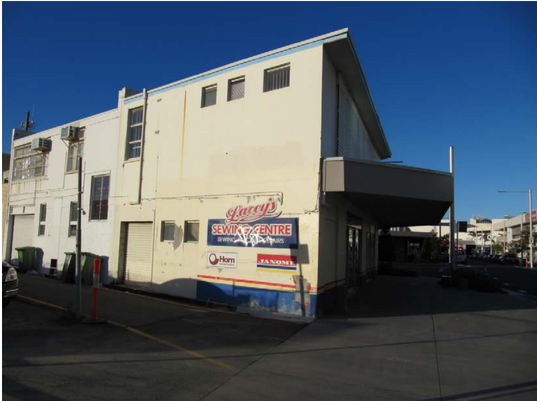
Figure 4.16 – Example of outdated building facades and graffiti
