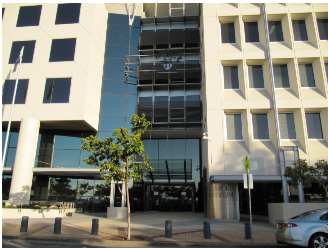
Figure 4.20 – The Courthouse with bollards in front
