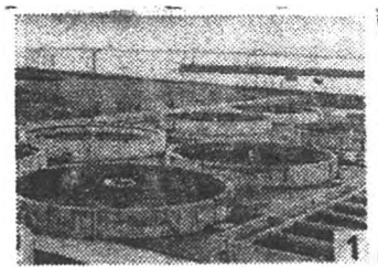
The round cement tank for rearing the adult milkfish (8.25 m in diameter, 1.5 m in depth)
