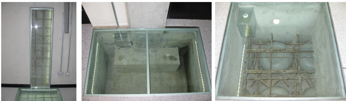
Figure 2 – Visual teaching tools (a) Recesses in a concrete wall showing exposed arrangement of reinforcement and glass panel to show build up of ground floor slab and finishes, (b) Pile cap foundations, (c) Void form flat slab system.
