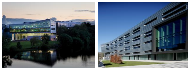
Fig. 1: The new Engineering building at the National University of Ireland Galway.
