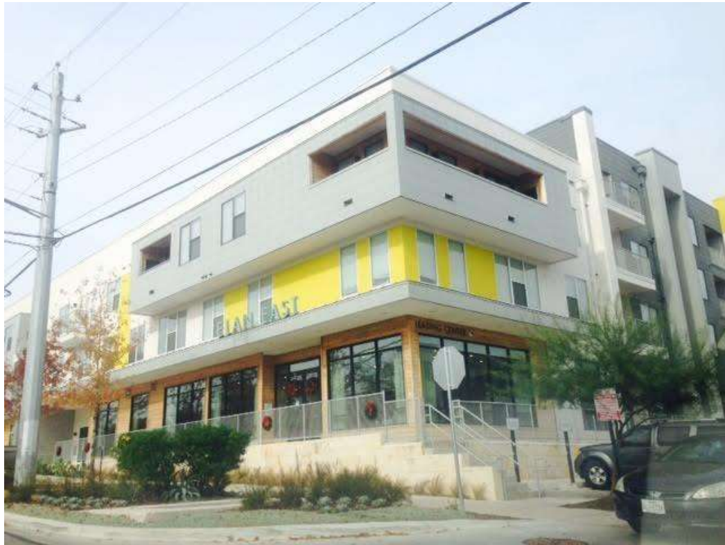
Figure 8: Elan East. Lofts on Manor Road constructed by Greystar Properties in partnership with Big Red Dog engineering. The website for the development reads, “Boutique-style living has never looked so good. With a fresh, modern take on apartment living, meet Elan East —Austin's newest address.” November 2015, Source: Author
