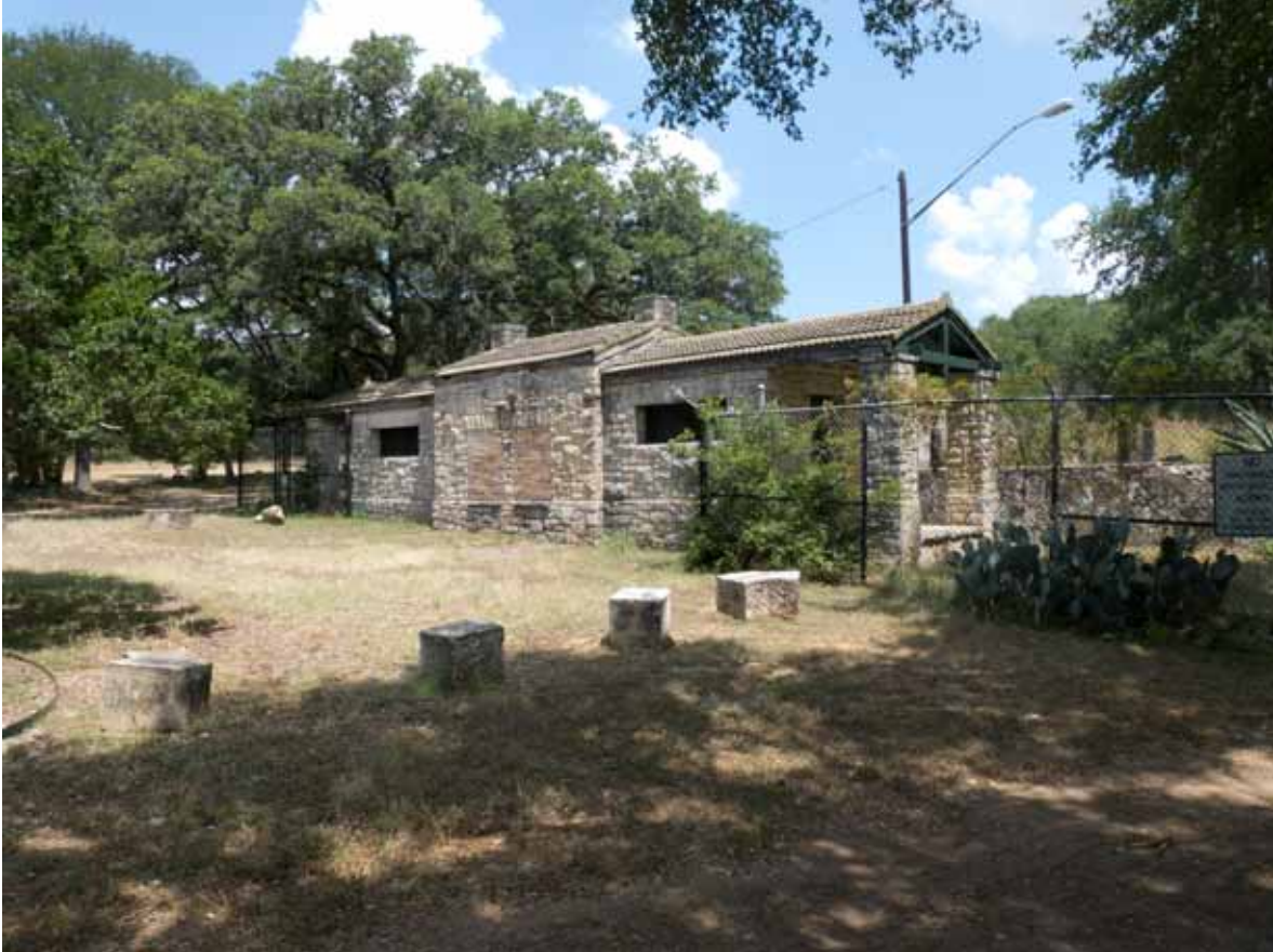
Landscape Characteristic F8 – Pistol/Skeet Range and Concession Building: South elevation of the concession building. Facing northwest.
