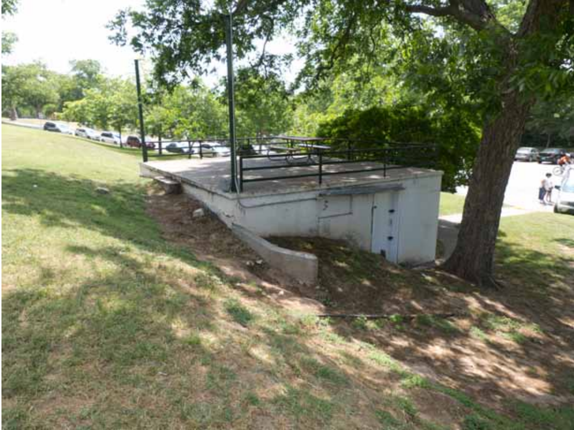
Landscape Characteristic F15 – Bandstand: Overview of bandstand building. North and west elevations, facing southeast.
