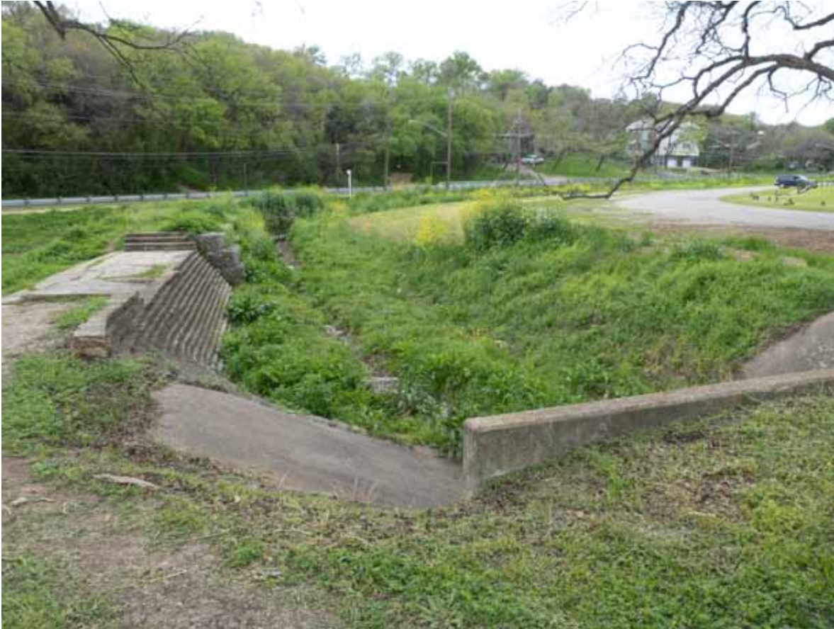
Landscape Characteristic F32 – Detention Pond/Swale: View of drainage swale and detention pond masonry check dam located just north of Robert E. Lee Road. Facing south. Photograph take by Julie McGilvray, 2012.
