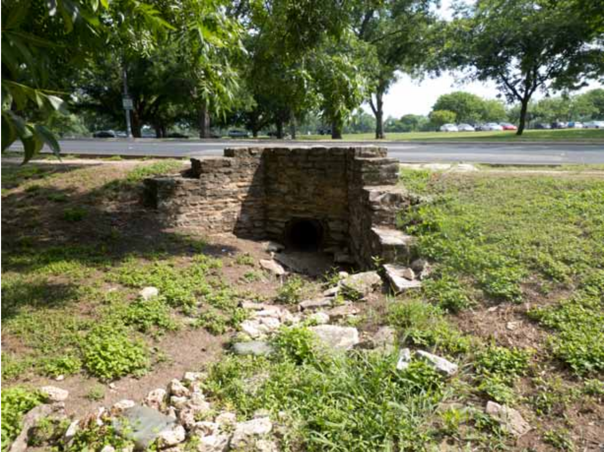
Landscape Characteristic E5 – Water Drainage System: Barton Springs Road culvert headwall. Located on the southwest side of Barton Springs Road, facing north. Photograph take by Julie McGilvray, 2012.
