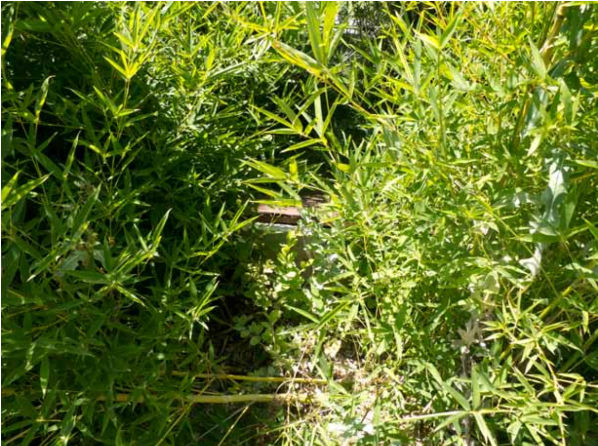
Landscape Characteristic F25 – Zilker Caretaker's Lodge Fallout Shelter: View of entry. Located on the north side of the lodge, within the side yard. Facing north.
