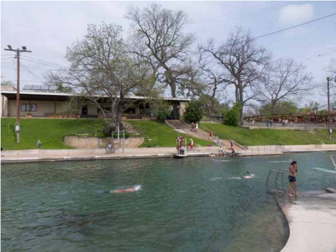
Landscape Characteristic F18 – Barton Springs Bath House: Overview of the eastern side of the south elevation, Barton Springs, and concession area (right side). Facing north-northeast. Photograph taken by Julie McGilvray, 2012.
