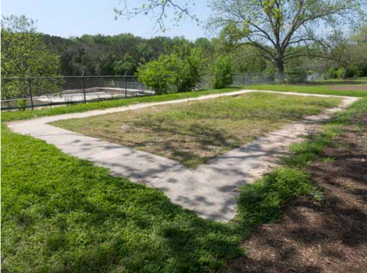
Landscape Characteristic F17 – Sand Pit (Wading Pool): Overview of concrete pool edge (now filled with sand and grasses). Located on the west side of the Barton Springs Bath House, facing southwest. Photograph take by Julie McGilvray, 2012.
