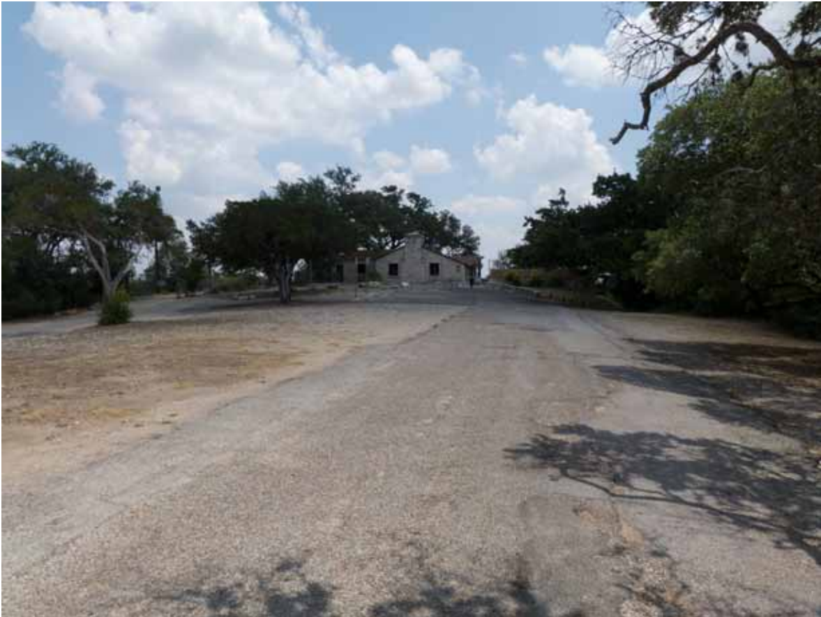
Landscape Characteristic B6 – Zilker Club House Zone: Overview of Club House and parking area. Facing northeast.
