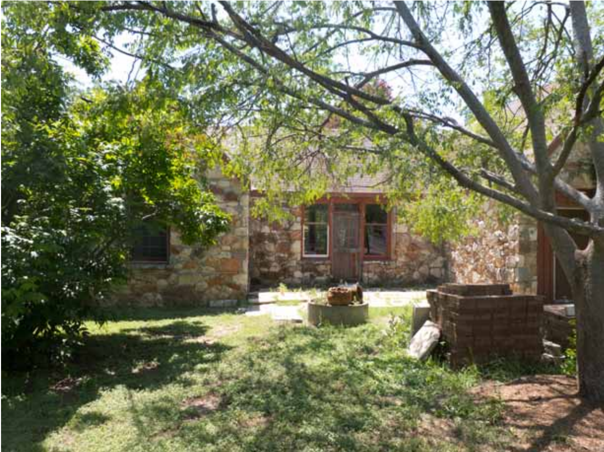
Landscape Characteristic F24 – Zilker Caretaker's Lodge: East elevation, facing west. Photograph take by Julie McGilvray, 2012.
