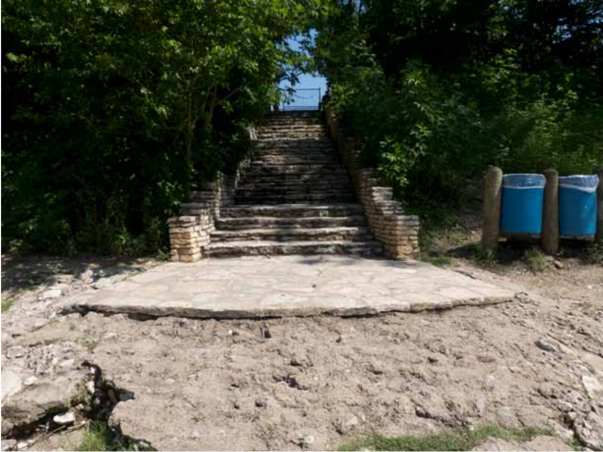
Landscape Characteristic F22 – Barton Creek Swimming Area: Masonry steps leading from the Barton Springs parking area to the lower Barton Creek area. Facing north. Photograph take by Julie McGilvray, 2012.
