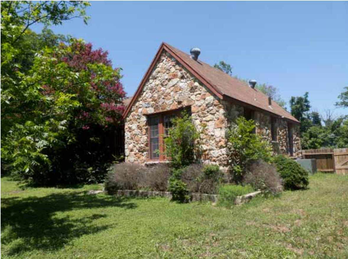
Landscape Characteristic F24 – Zilker Caretaker's Lodge: West and south elevations. Facing northeast. Photograph take by Julie McGilvray, 2012.
