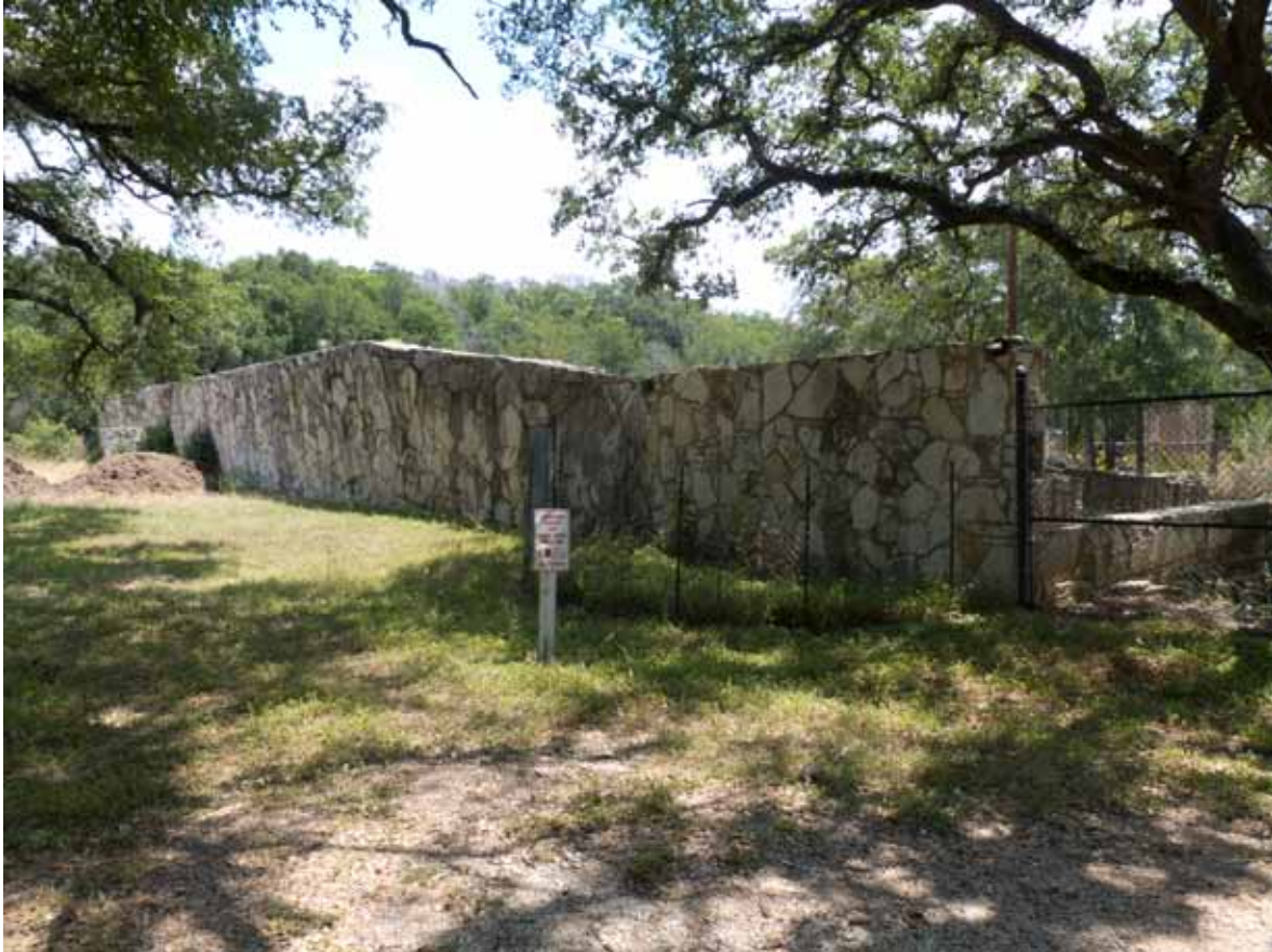
Landscape Characteristic F8 – Pistol/Skeet Range and Concession Building: East elevation of the range wall. Facing northeast.
