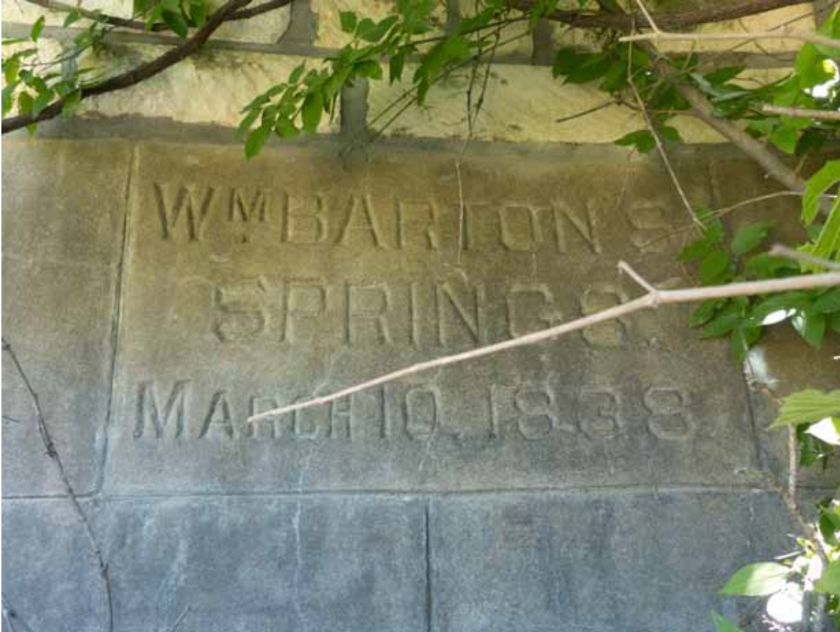
Landscape Characteristic F31 – Elk’s Pit (Eliza Spring): William Barton’s Spring concrete panel. Located on wall panel of pit. Facing east.
