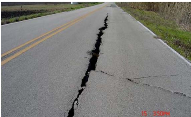
Left: Photo of pavement cracks in a new Austin subdivision in 2009. Right: Longitudinal cracking on Golden Falls Drive in Travis County in 2008. Photo credit: City of Austin.
