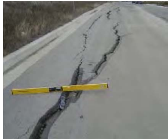
Left: Photo of pavement cracks in a new Austin subdivision in 2009. Right: Longitudinal cracking on Golden Falls Drive in Travis County in 2008. Photo credit: City of Austin.
