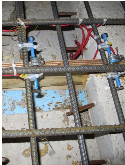
Figure 3.11: Gages Secured to Reinforcement
