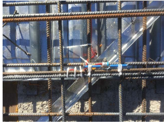
Figure 3.31: Gage at the Edge of Girder
