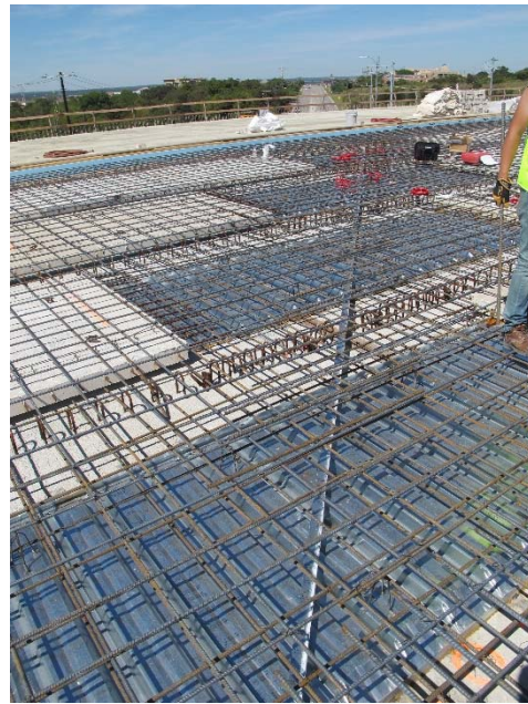
Figure 3.28: Reinforcement over the PMDF
