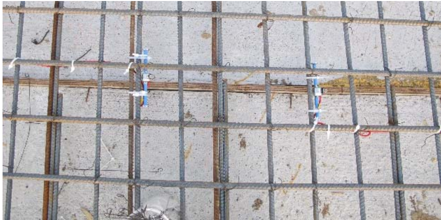
Figure 3.44: Top Layer Gages over the Crack Former
