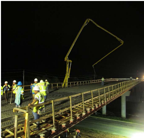
Figure 3.15: Concrete Pump Truck
