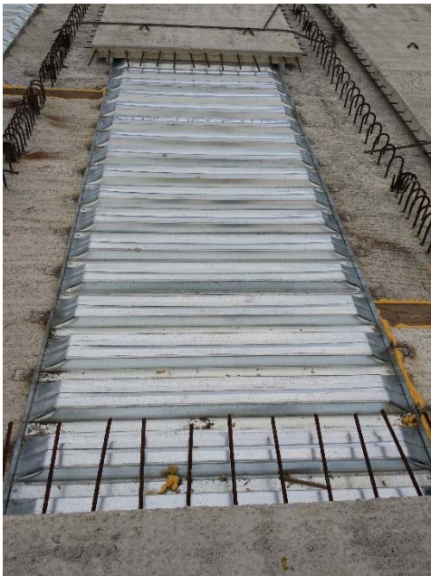
Figure 3.27: Permanent Metal Deck Form
