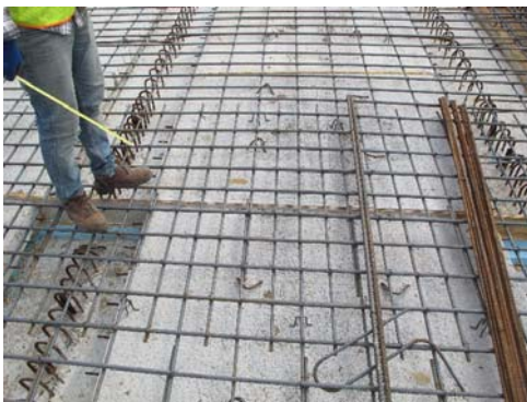
Figure 3.40: Additional Reinforcement
