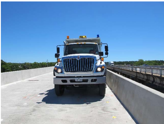
Figure 3.52: Exterior Girder Position
