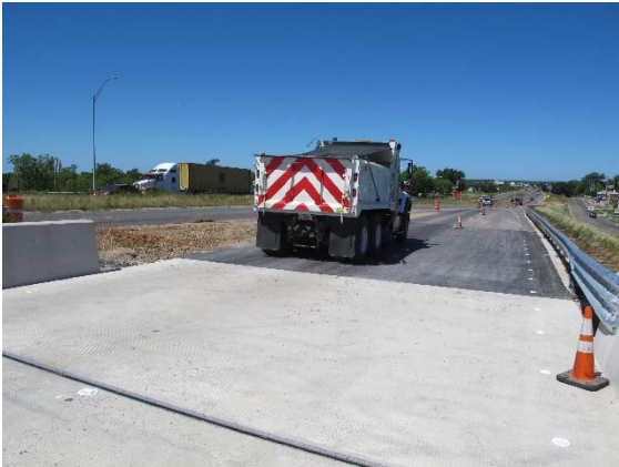
Figure 3.50: Removal of Truck from Span
