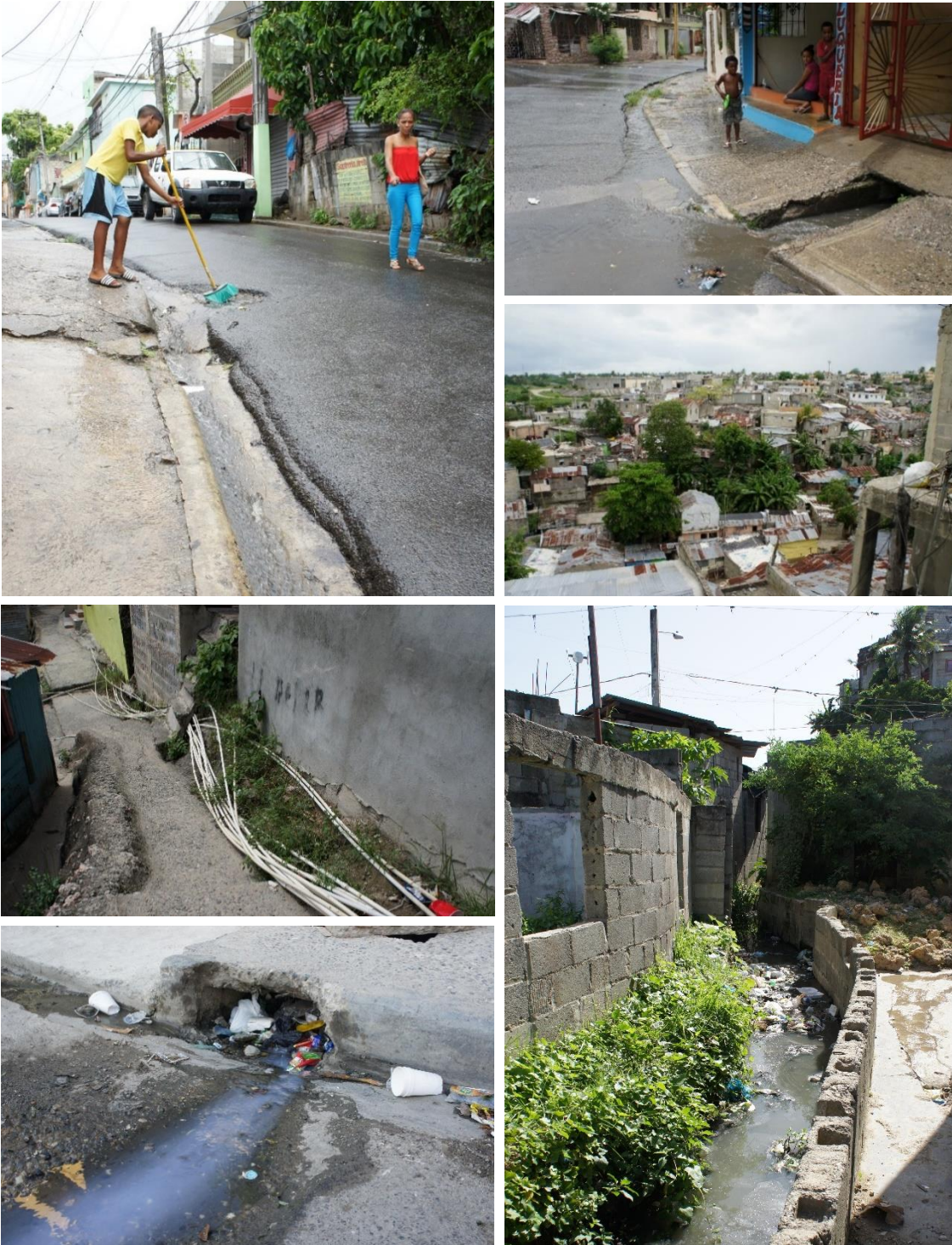
Figure 2 Stormwater Management in Los Platanitos. Clockwise from top left: a) A child sweeps runoff from Hermanas Mirabal to an inlet that drains to the channel. b) An inlet to the channel. c) High levels of impervious cover. d) Trash accumulations in the channel frequently block the free-flow of water. e) Trash and contaminated water is carried into an inlet that drains to the channel. f) Illegal connections to the household water system. Photographs by Kelly Strickler.
