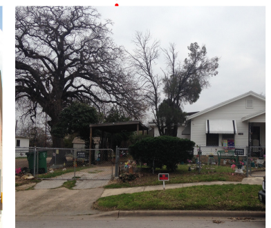
Uneven paved surfaces
