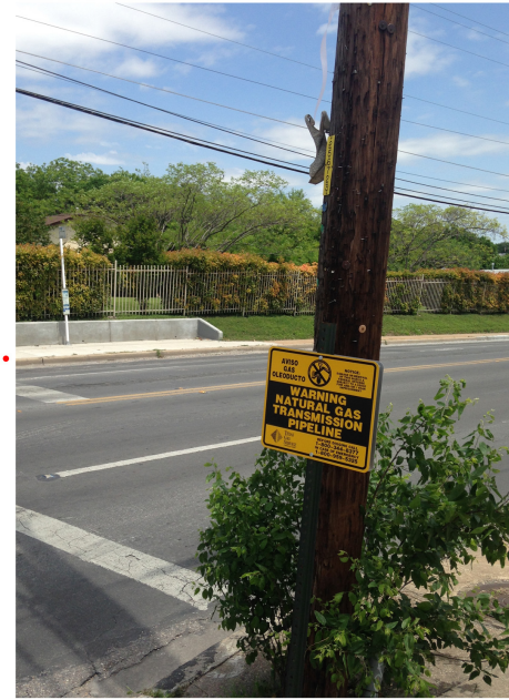
Gas pipe line warning
