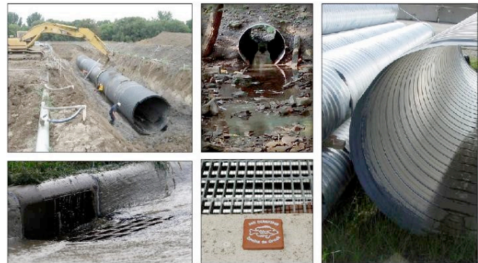
Above: Assorted components of modern stormwater drainage management systems. Sources: See Photo Index.
