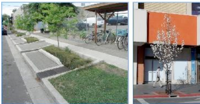
Top: A drainage pipe from a roof directs stormwater onto an impervious street. Bottom Left: Bioswales with curb cuts allow for runoff to be naturally filtrated. Bottom Right: A tree box filter. Sources: See Photo Index.
