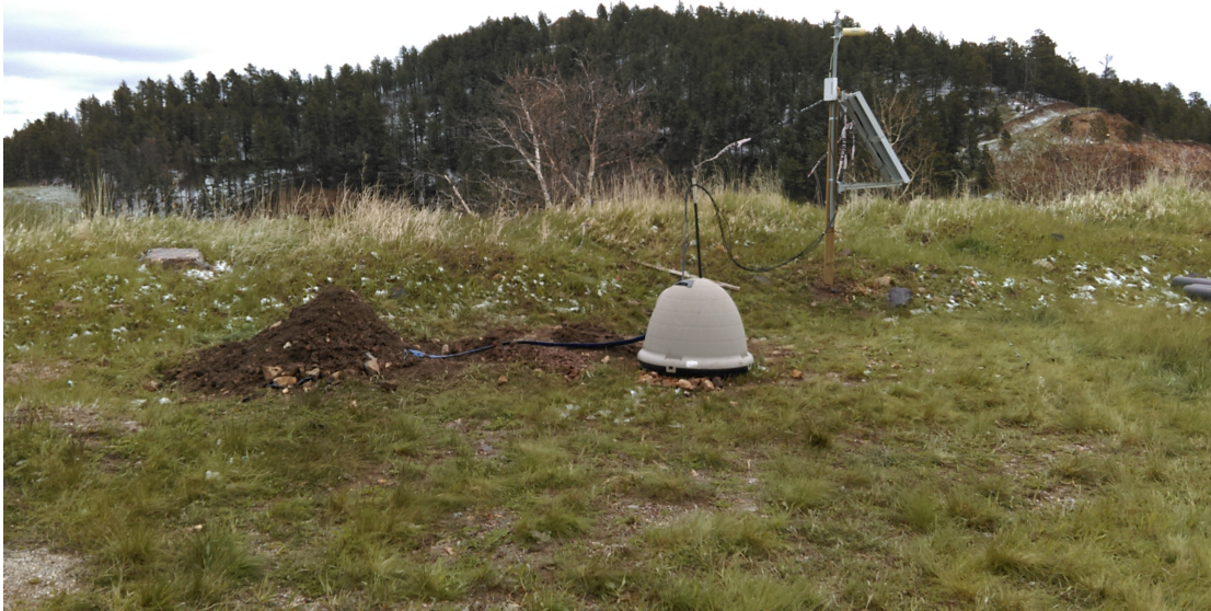
Figure 6.7: An example of a surface station (RRDG) after it is completed. Note the dog house where electronics are stored, the solar panels, the radio on the pole, and the GPS antenna above the radio (the small hemispherical object on top of the pole). A single cable, reinforced to protect against rodents, was run from the electronics house to the seismometer enclosure.
