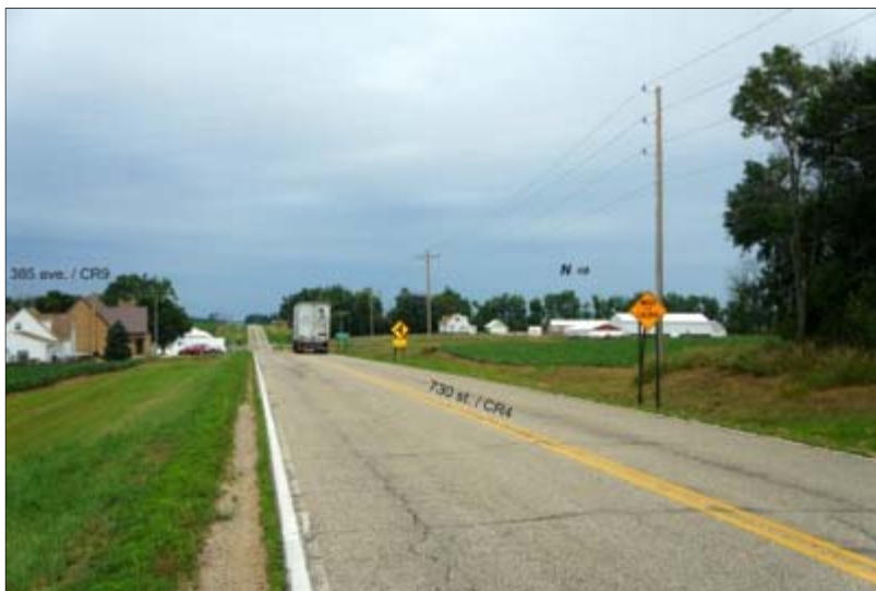
Figure 11: Ground view of intersection of County Roads 4 and 9, Jackson County.
