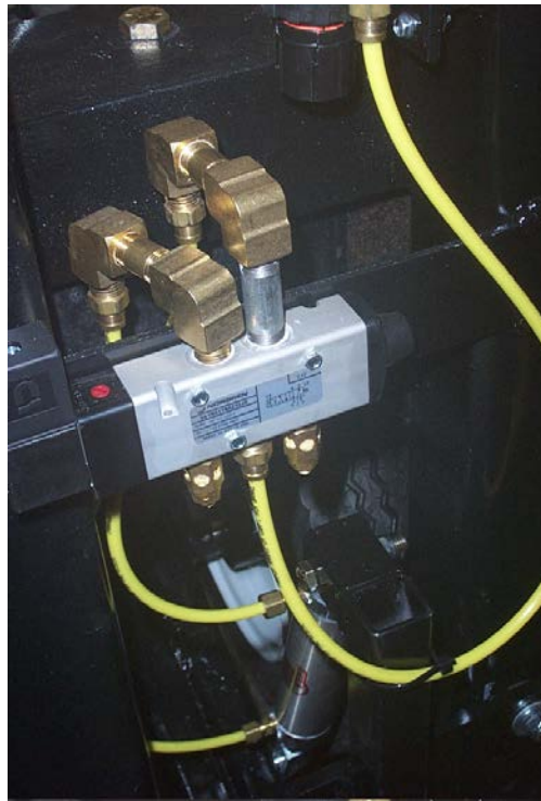
Figure 16: Pneumatic valve with a supply line from a pressure regulator at the top of the picture controlling the cylinder that raises and lowers the friction wheel near the bottom of the picture.
