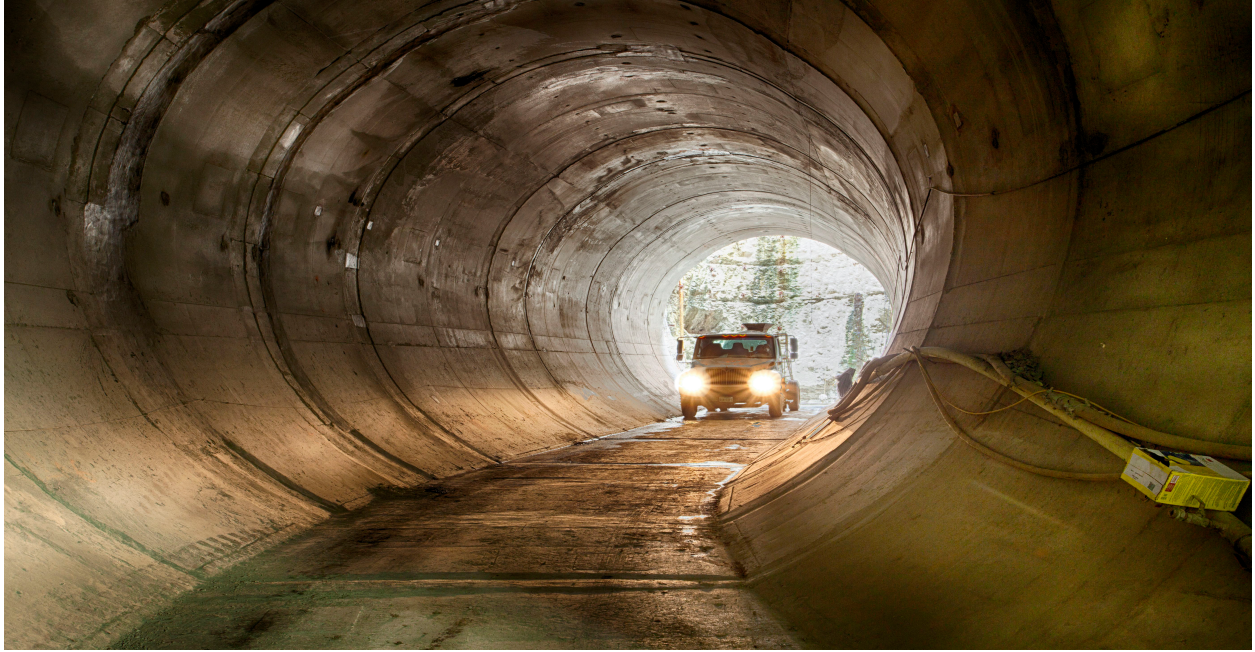
4 th Street Connector Tunnel
