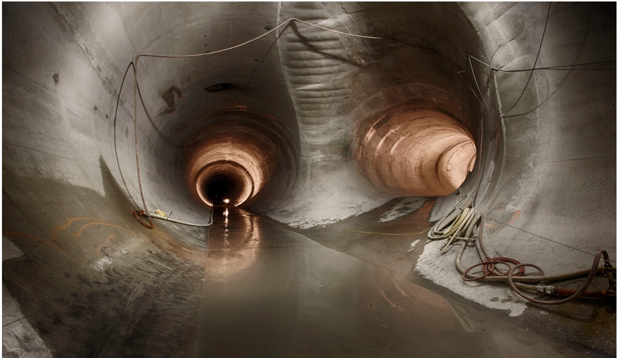
Confluence Main & 4 th St Connector Tunnel
