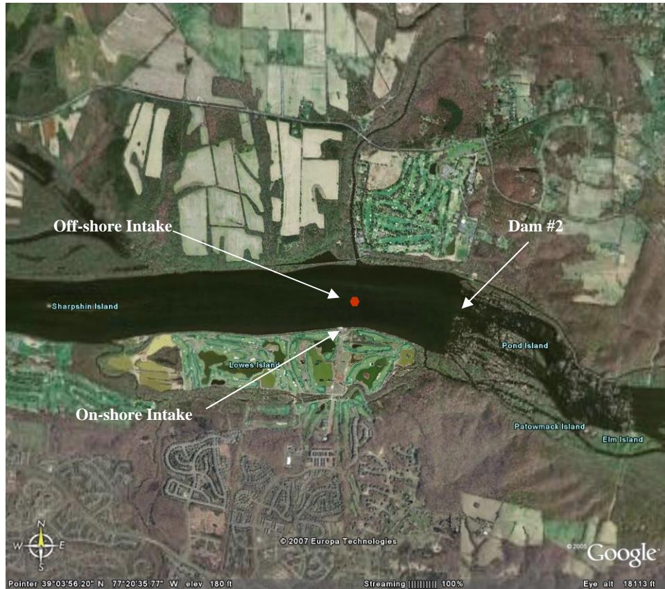
Figure 1.1. Aerial photo of the Potomac River and the approximate location of the off-shore intake in the Seneca Pool.
