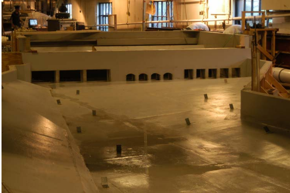
Figure 4. View of the model gate house from downstream.
