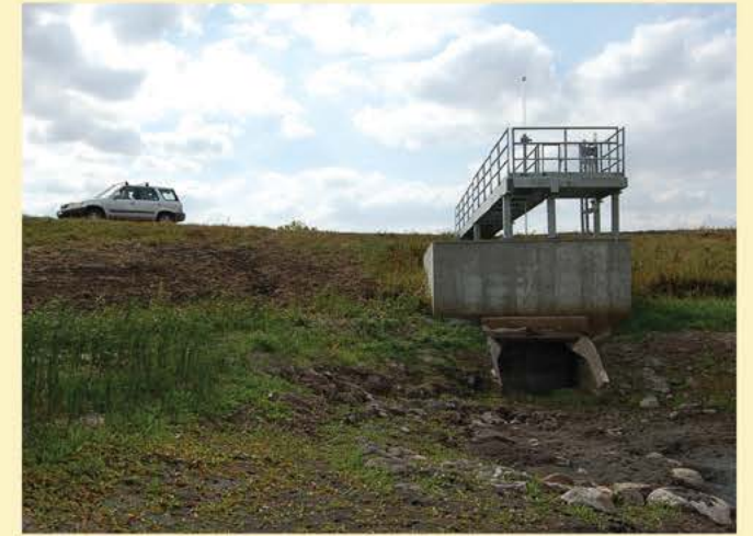
Water levels in the impoundments are regulated by control gates like this one. © Center for Changing Landscapes.
