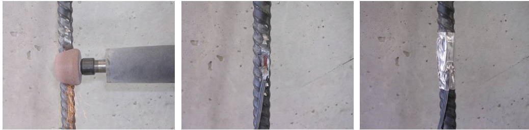
Figure 3-21. Installation of strain gauge for measuring steel strains.
