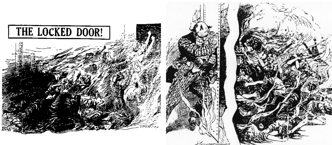
Figure 12: Two political cartoons depicting the locked door of the ninth floor during the Triangle factory fire, 1911. Both images are part of the Triangle collection at the Kheel Center for Labor-Management Documentation and Archives, M.P. Catherwood Library, Cornell University.
