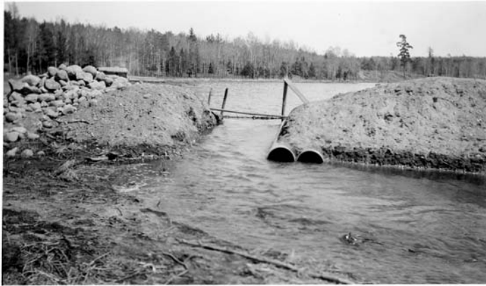
ITASCA STATE PARK.SP.#.1.LAKE ITASCA MINNESOTA,MAY 11 1934. (PROJECT.#.50.) THE MISSISSIPPI RIVER AS IT LEAVES LAKE ITASCA, THE EARTHEN DYKE AND TEMPORARY OUTLET.
