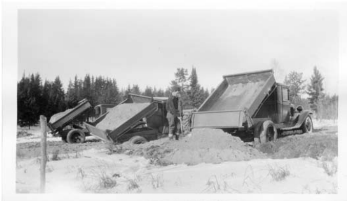
PHOTO #62 PROJECT # 48 JOB # 4 Filling banks of Mississippi River, vicinity Beaver Dam.
