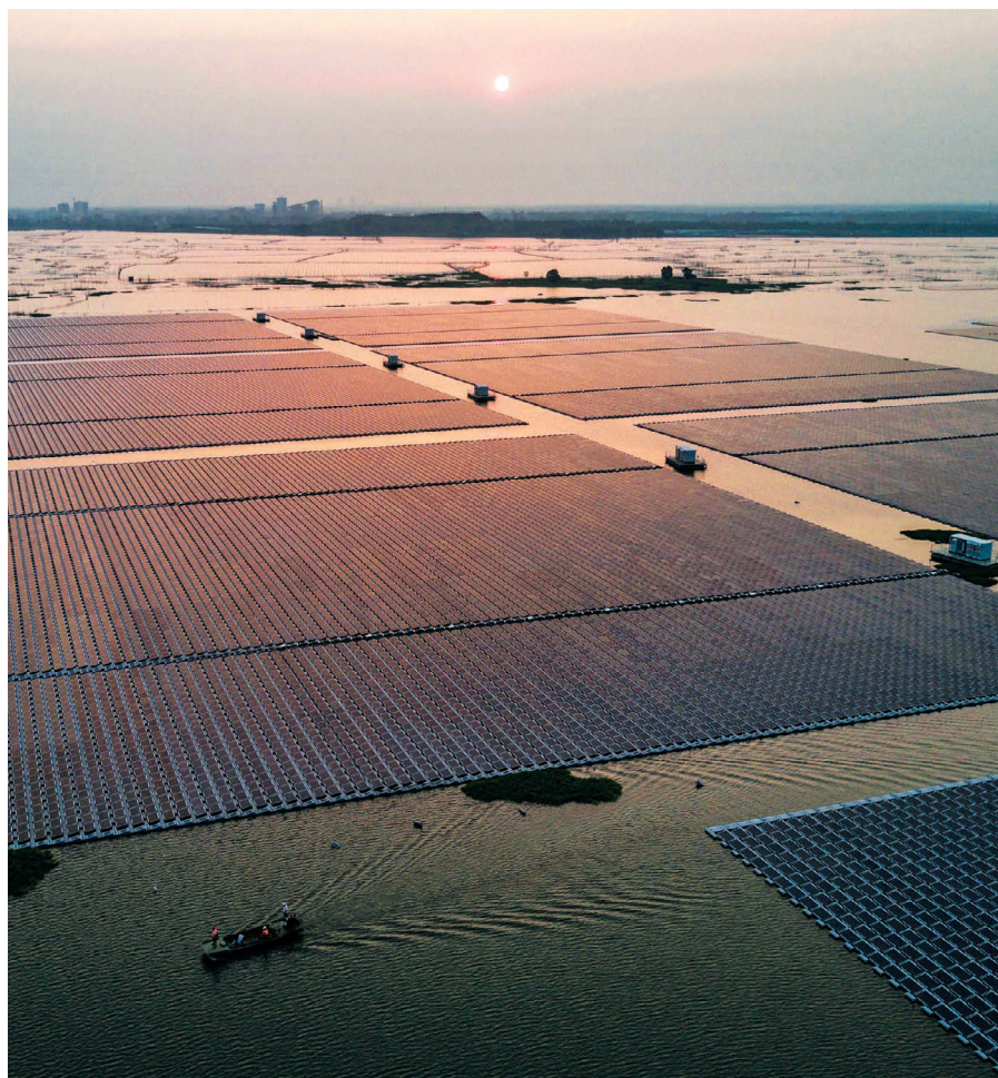
A solar farm floats on a lake that formed after the collapse of a deep coal mine in Huainan, China.
