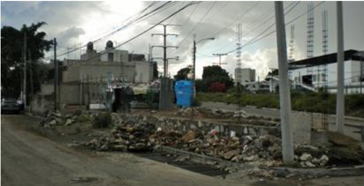
Illustration 17: The construction of Guadalajara's shelter. Photo taken during the summer of 2014.
