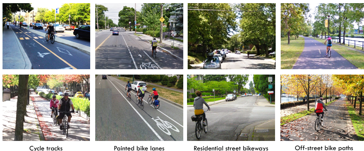
Figure 1: Examples of the four bikeway types examined, top row in Montréal, bottom row in Vancouver (photo credits: authors, Ken Ohrn, Google Streetview)
