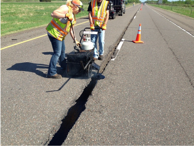
Figure 3.52 Filling Longitudinal Crack with Mastic.
