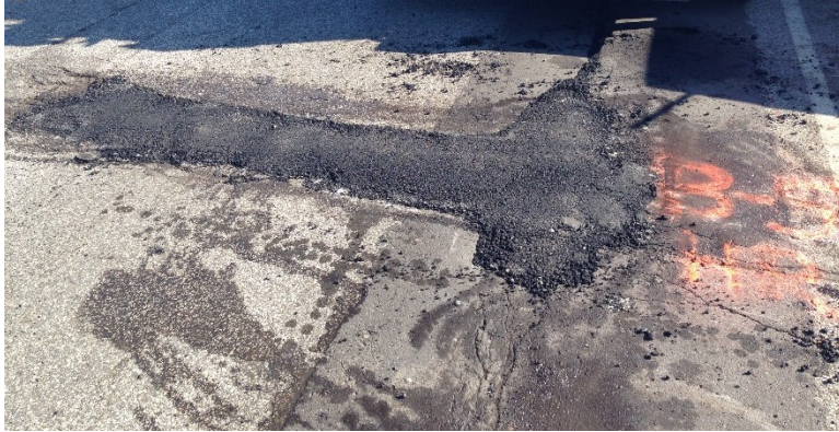
Figure 3.34 Pothole B-5 after Patching.
