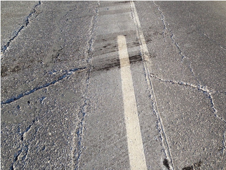
Figure 3.83 Pothole E-4 (119 Days after Installation).
