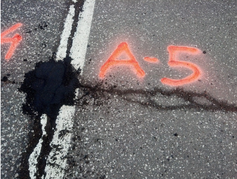
Figure 3.10 Pothole A-5 after Patching.
