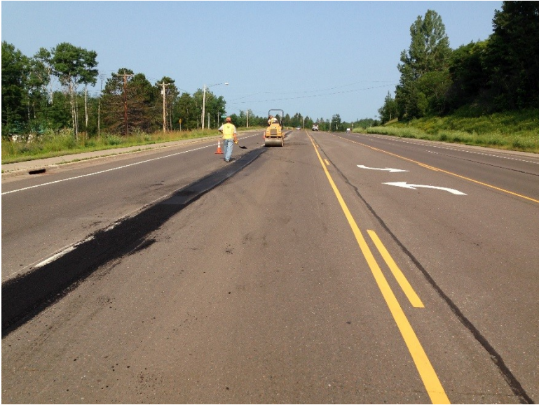
Figure B13: Mill and Fill Step 4.
