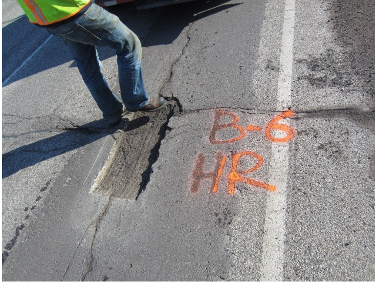
Figure 3.31 Pothole B-6 after Milling.
