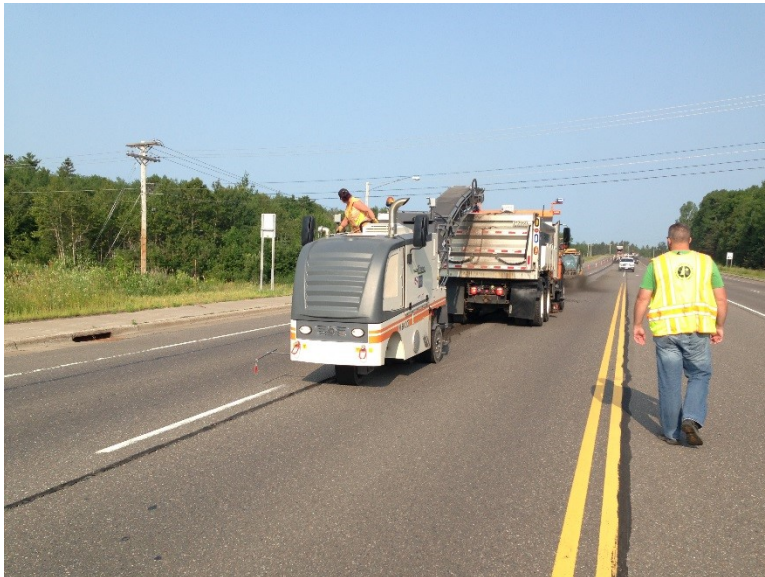
Figure B9: Mill and Fill Step 1.
