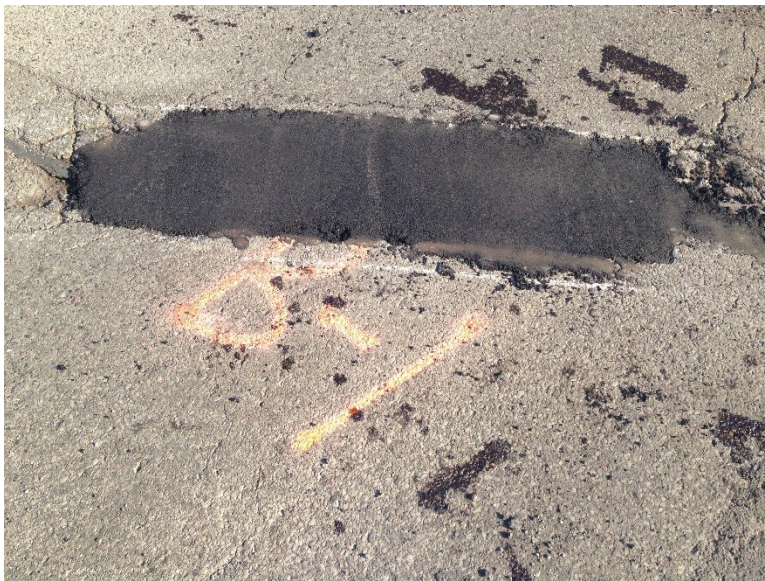
Figure 3.36 Pothole B-1 after Patching.
