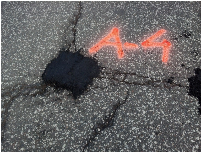
Figure 3.14 Pothole A-4 after Patching.
