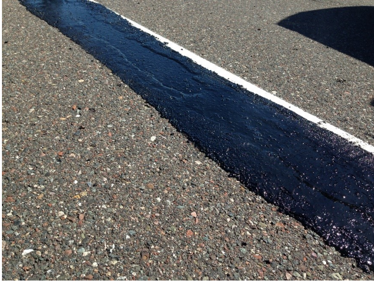
Figure 3.54 Finished Mastic Patch.
