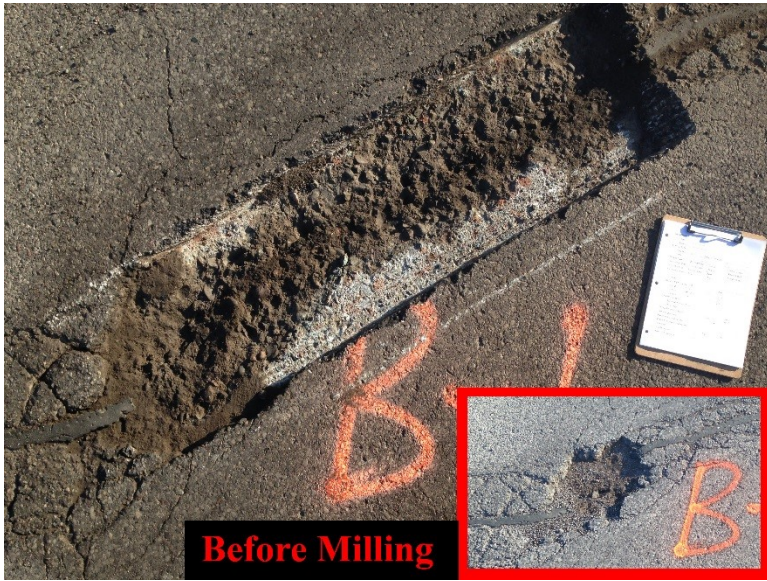
Figure 3.25 Pothole B-1 before and after Milling.
