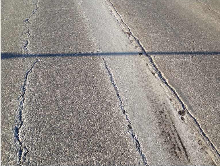
Figure 3.84 Pothole E-5 (119 Days after Installation).
