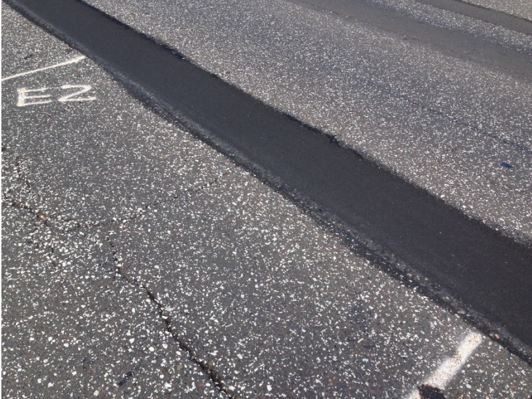
Figure 3.78 Pothole E-2 (28 Days after Patching).
