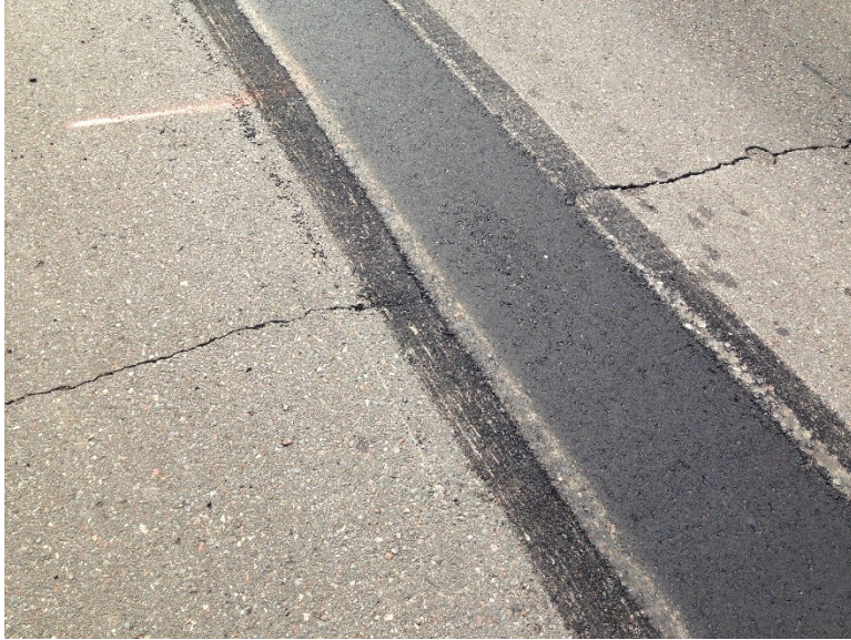
Figure 3.61 Pothole D-3 with Clean Compaction.
