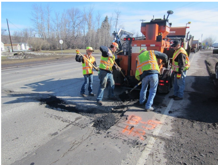
Figure B7: Hot Recycler Step 4.
