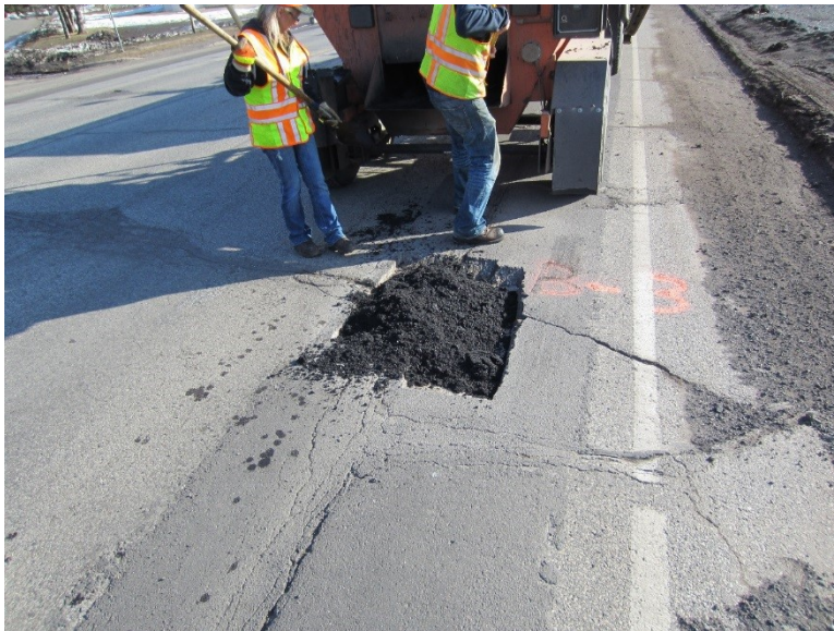
Figure B3: Cold Mix Step 3.
