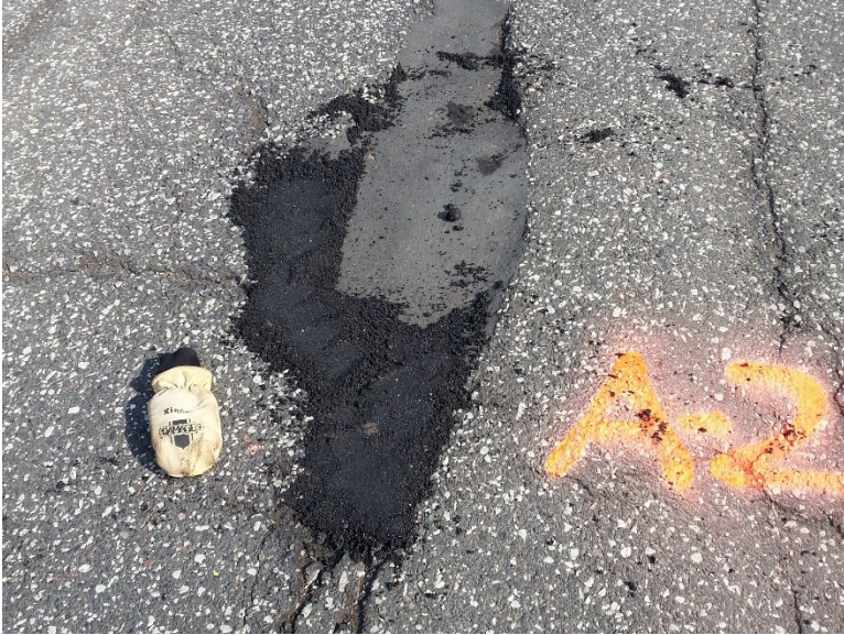
Figure 3.7 Pothole A-2 after Patching.
