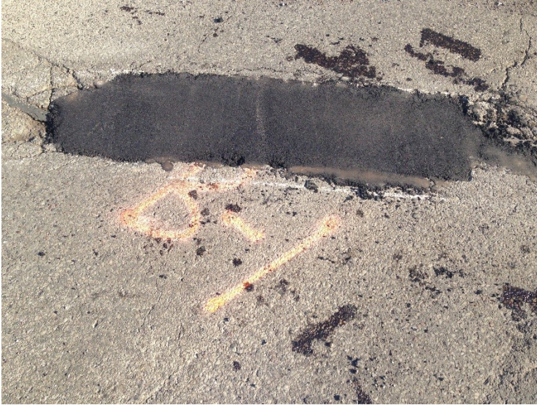
Figure 3.32 Pothole B-1 after Patching.
