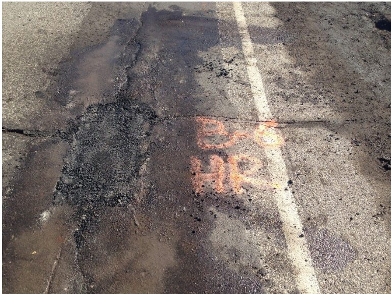
Figure 3.35 Pothole B-6 after Patching.
