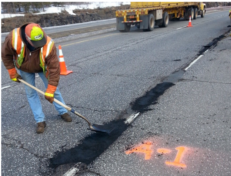
Figure 3.6 Pothole A-1 after Patching.
