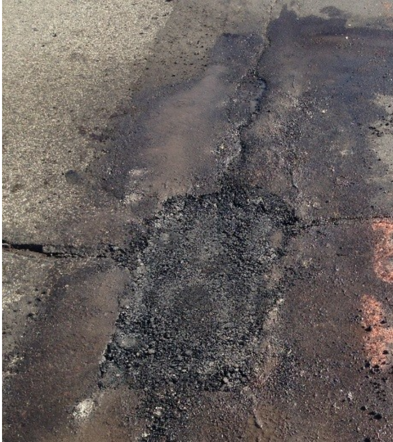
Figure 3.45 Pothole B-6 immediately after Patching.
