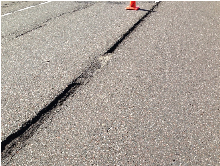
Figure 3.51 Longitudinal Crack before Placing Mastic (Cleaned with Compressed Air).
