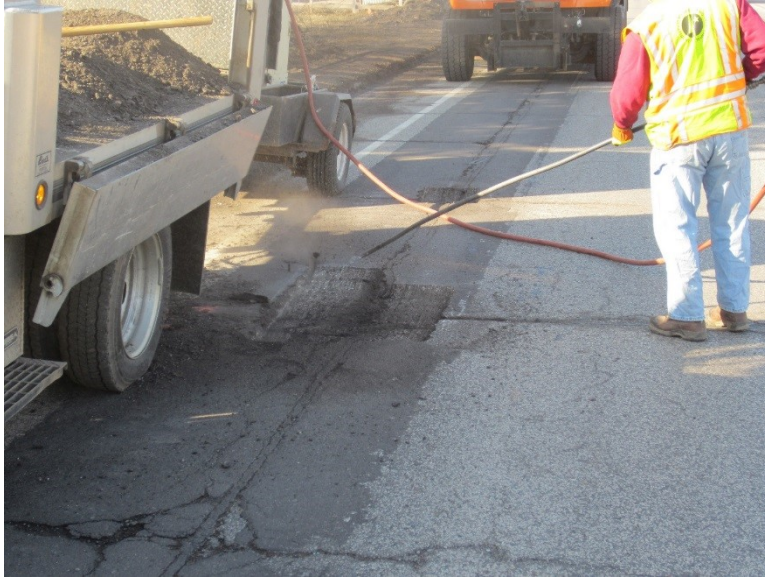
Figure B2: Cold Mix Step 2.
