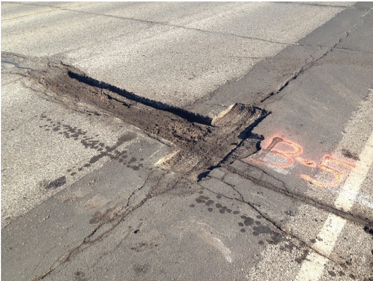
Figure 3.30 Pothole B-5 after Milling.
