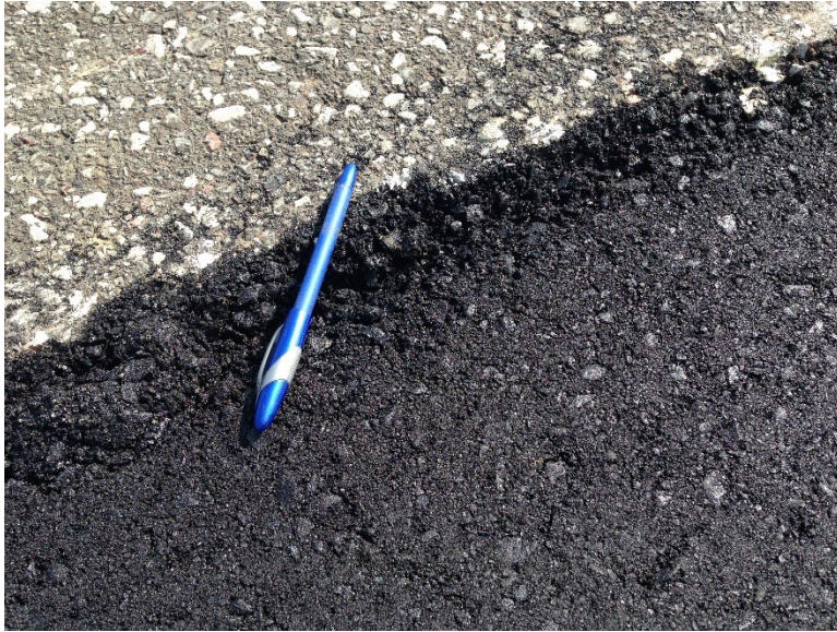
Figure 3.77 Lack of Compaction and Material near Interface of Patch Material and Roadway.
