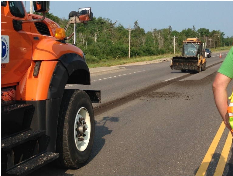
Figure B11: Mill and Fill Step 2.
