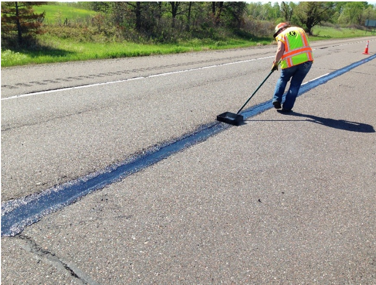
Figure 3.53 Using a Box Screed to Evenly Spread Mastic along Crack.
