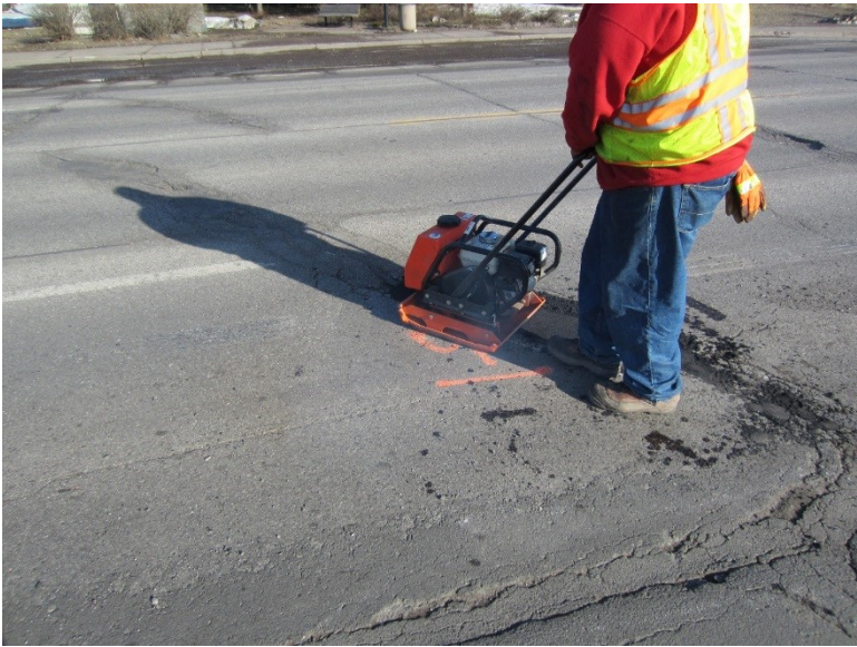
Figure B4: Cold Mix Step 4.
