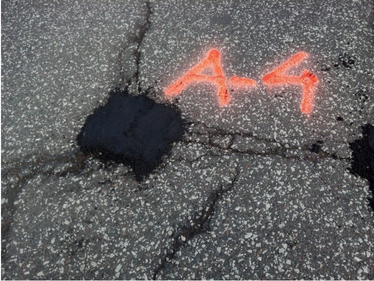
Figure 3.9 Pothole A-4 after Patching.
