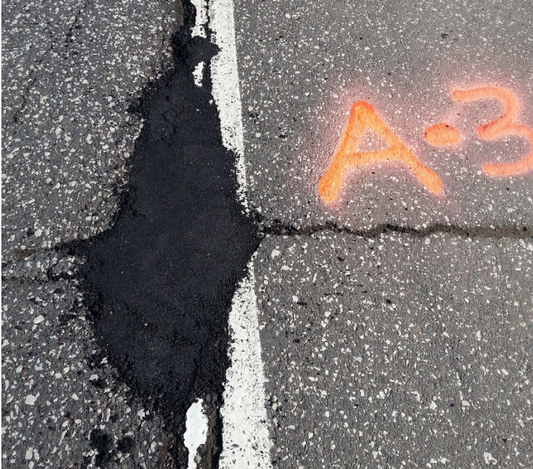
Figure 3.8 Pothole A-3 after Patching.
