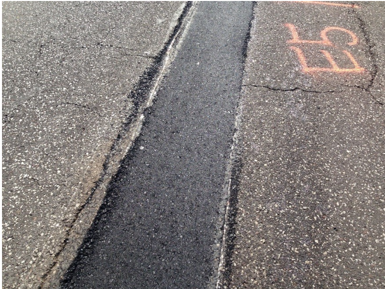
Figure 3.76 Pothole E-5 after Compaction.
