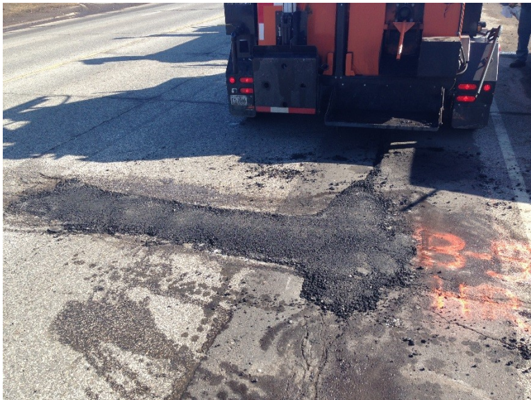
Figure 3.42 Pothole B-5 after Patching.
