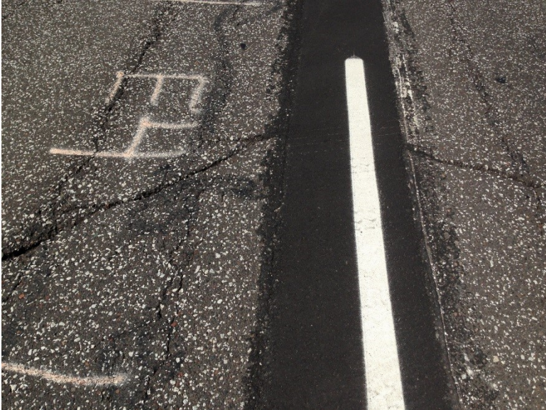
Figure 3.79 Pothole E-4 (28 Days after Patching).
