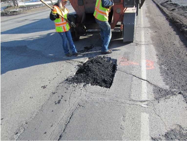
Figure 3.27 Pothole B-3 while Filling with Cold Mix Material.
