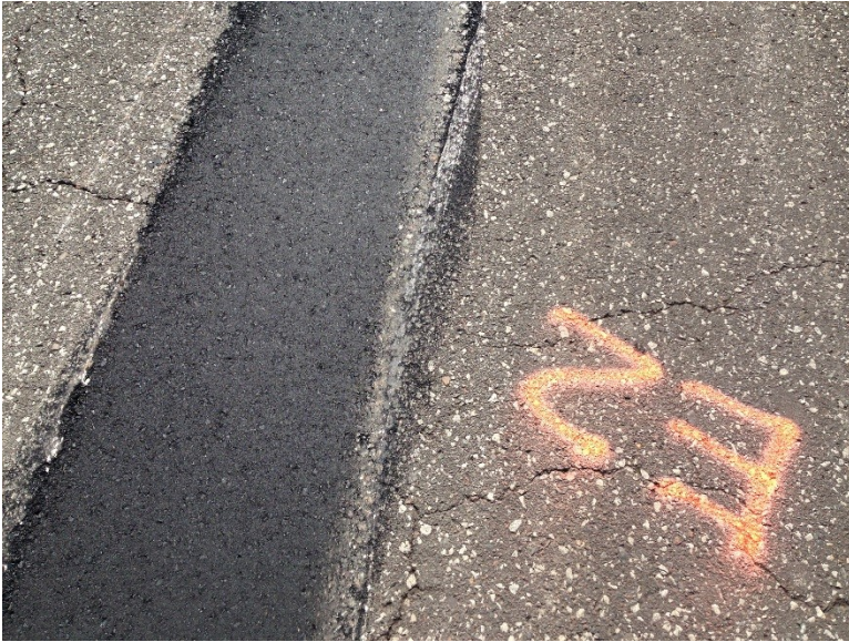
Figure 3.73 Pothole E-2 after Compaction.
