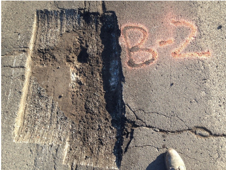
Figure 3.26 Pothole B-2 after Milling.
