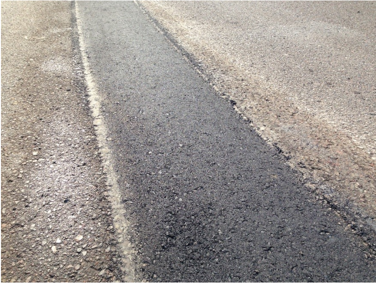
Figure 3.60 Pothole D-2 with Clean Compaction.
