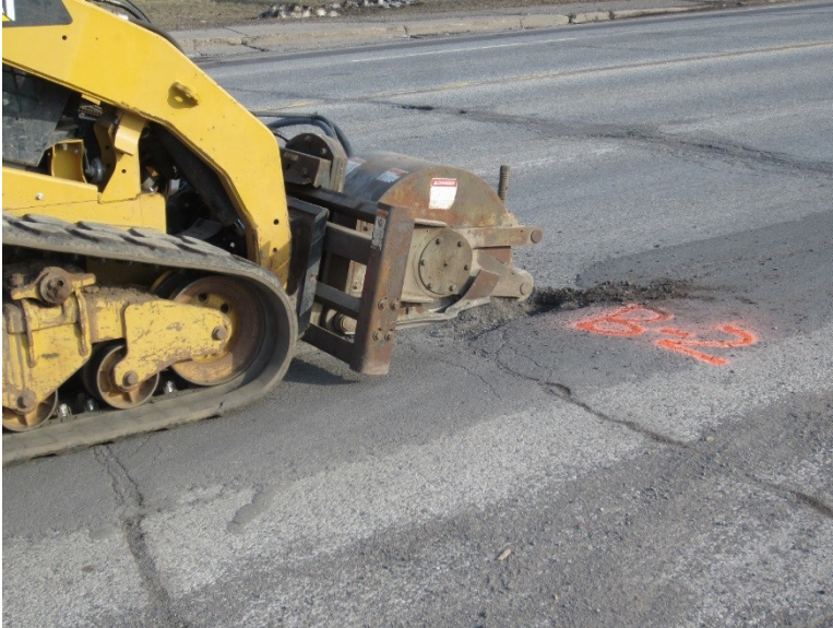
Figure B1: Cold Mix Step 1.
