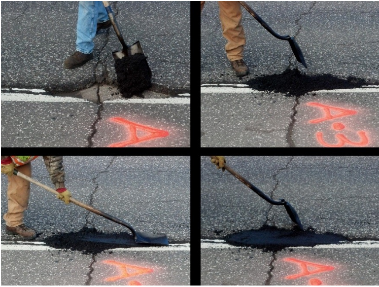
Figure B5: Cold Mix Placement and Compaction Using Only a Shovel.
