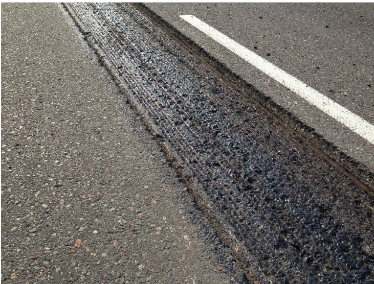
Figure 3.57 Milled Trench.
