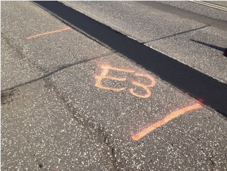
Figure 3.74 Pothole E-3 after Compaction.
