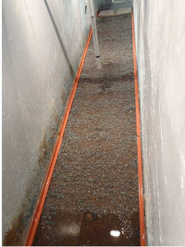
Figure 4.84. View looking upstream after six hours of run time. Almost all of the FRM has been washed away and the depression near the shoulder has gotten deeper.
