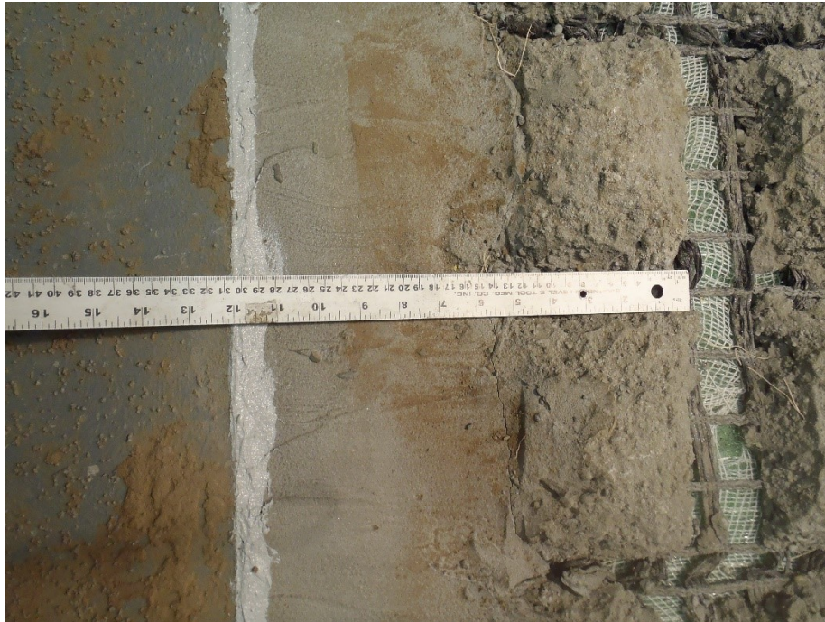
Figure 3.17. Flexamat® “paved” into the shoulder with Portland cement grout to transition onto the slope. Seam of paving and shoulder sealed with a polyurethane single component sealant (white). Flow is left to right in this image.
