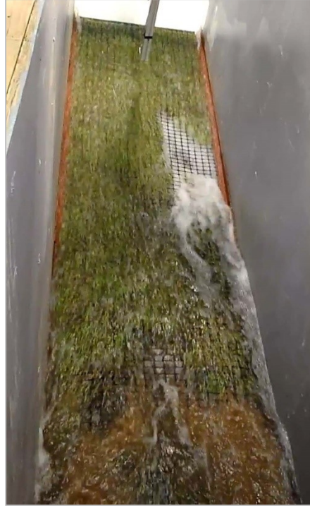
Figure 4.65. During final 4-5.5 hour run, catastrophic erosion took place. Most of the lower slope began eroding under the sod, which had come loose but was held from being washed away by the geogrid and staples.
