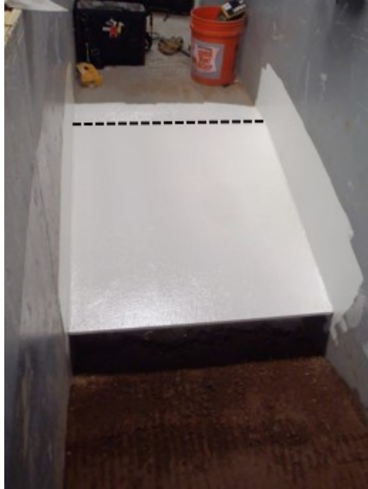
Figure 3.22. Simulated extended shoulder paving in the 4H:1V flume, prior to installation of stabilization materials. A dashed line has been added at the shoulder edge at the top of the slope.
