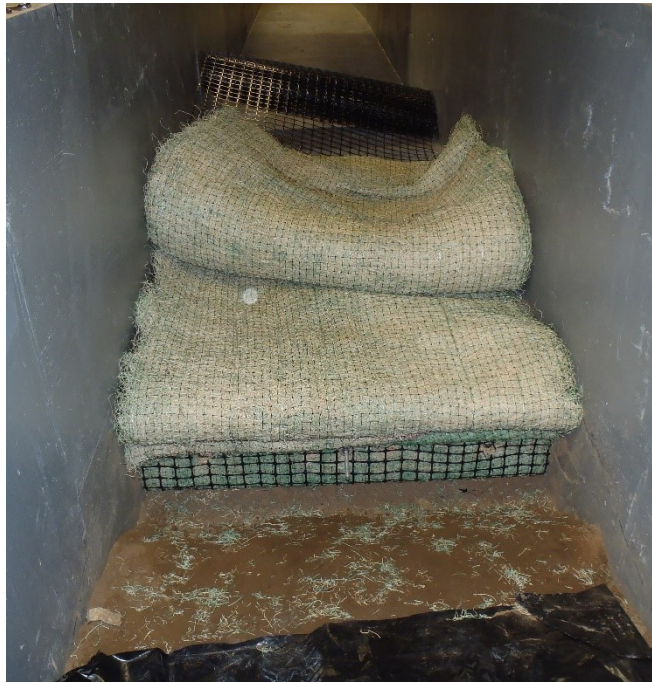
Figure 3.15. View looking upslope. Armored sod material wrapped around a piece of lumber and bolted to framing under the shoulder. Once backfilled with soil, the armored sod material on the shoulder would be flipped down to cover the slope.
