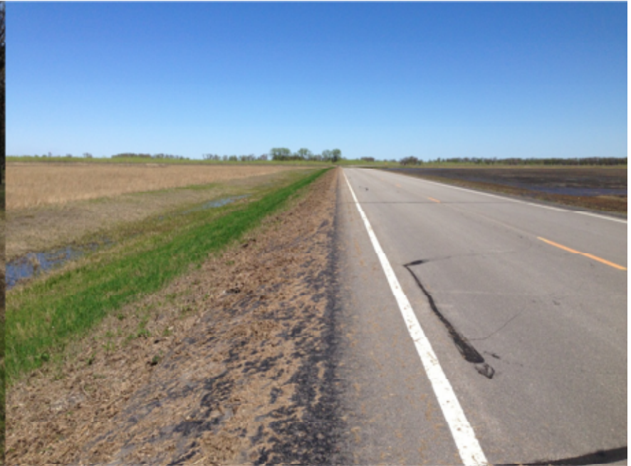
DOWNSTREAM LOOKING EAST
