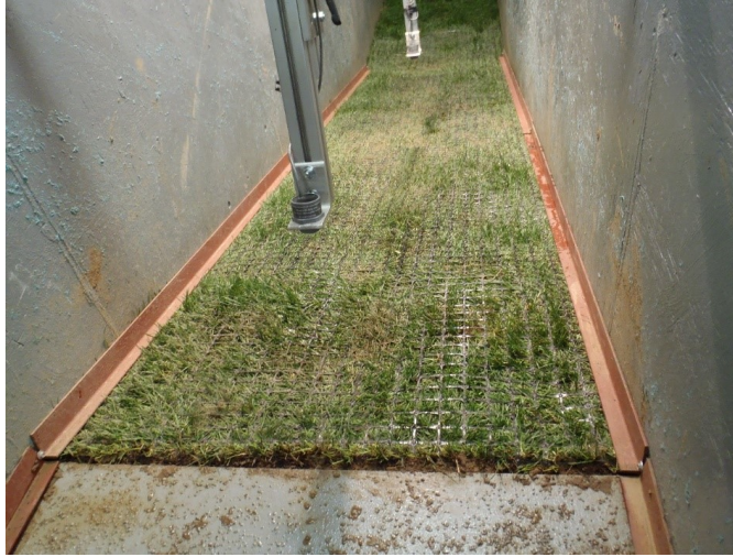
Figure 4.54. Looking downstream from shoulder. Installed sod and geogrid before testing.
