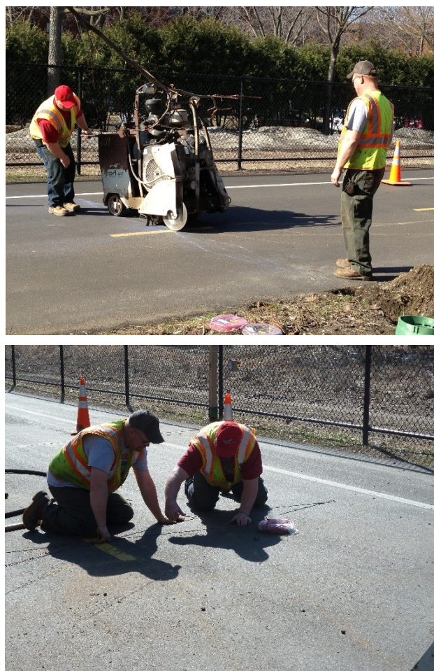
Figure 14: Installing an Inductive Loop in a Saw Cut on a Multi-purpose Path
