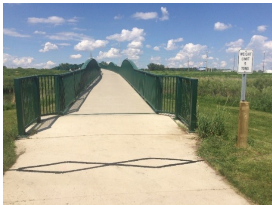
Figure 21: Infrared and Short Duration Inductive Loop Installation on Surface of a Shared-use Path
