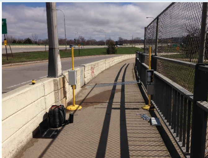
Figure 13: Microwave Detector Installation using Stanchions
