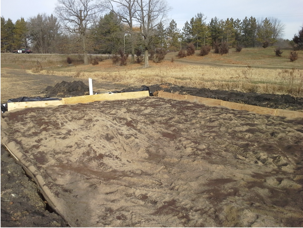
Figure 33. Construction: iron aggregate spread across sand layer
