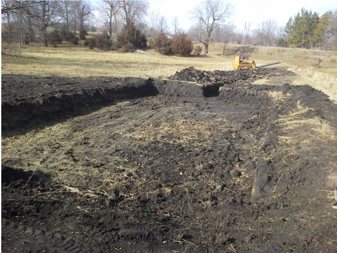
Figure 31. Construction: Excavation complete.
