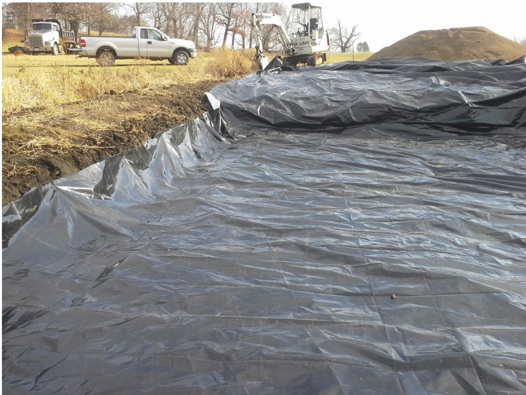
Figure 32. Construction: Impermeable liner.
