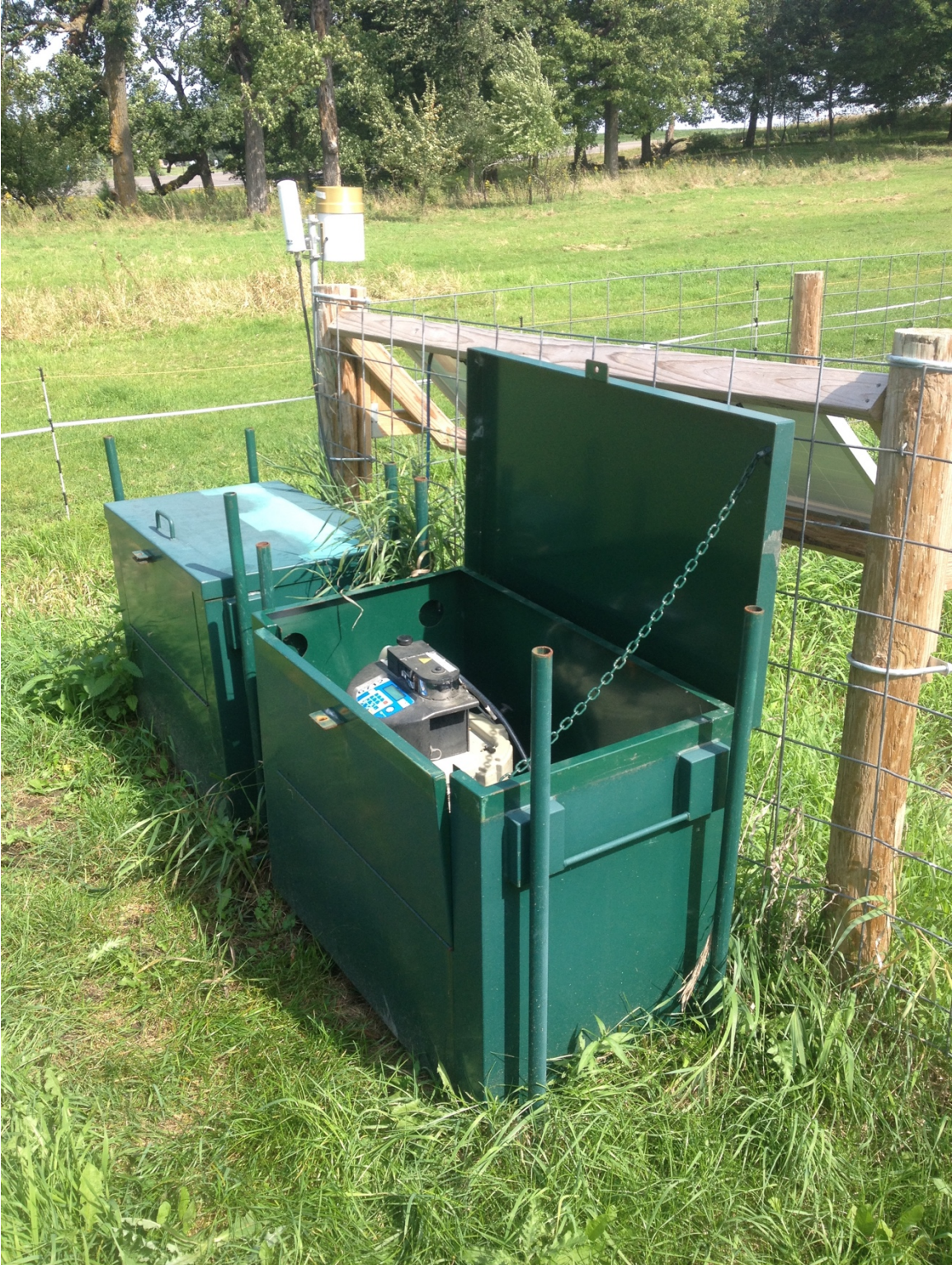
Figure 35. Monitoring: Protective (green) cabinets holding monitoring equipment (ISCO 6712 automatic water sampler visible).
