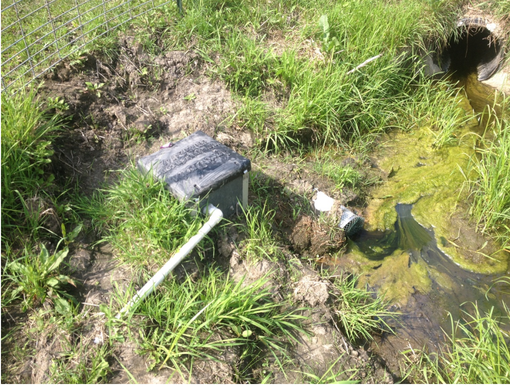
Figure 38. Monitoring: Agri Drain Inline Water Level Control Structure™ (black lid).
