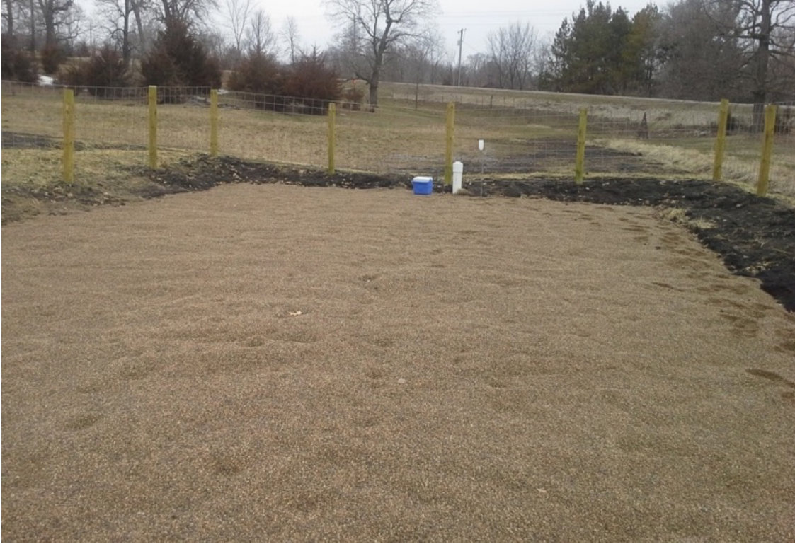
Figure 5. Site photo of Iron Enhanced Sand Filter (IESF) shortly after construction.
