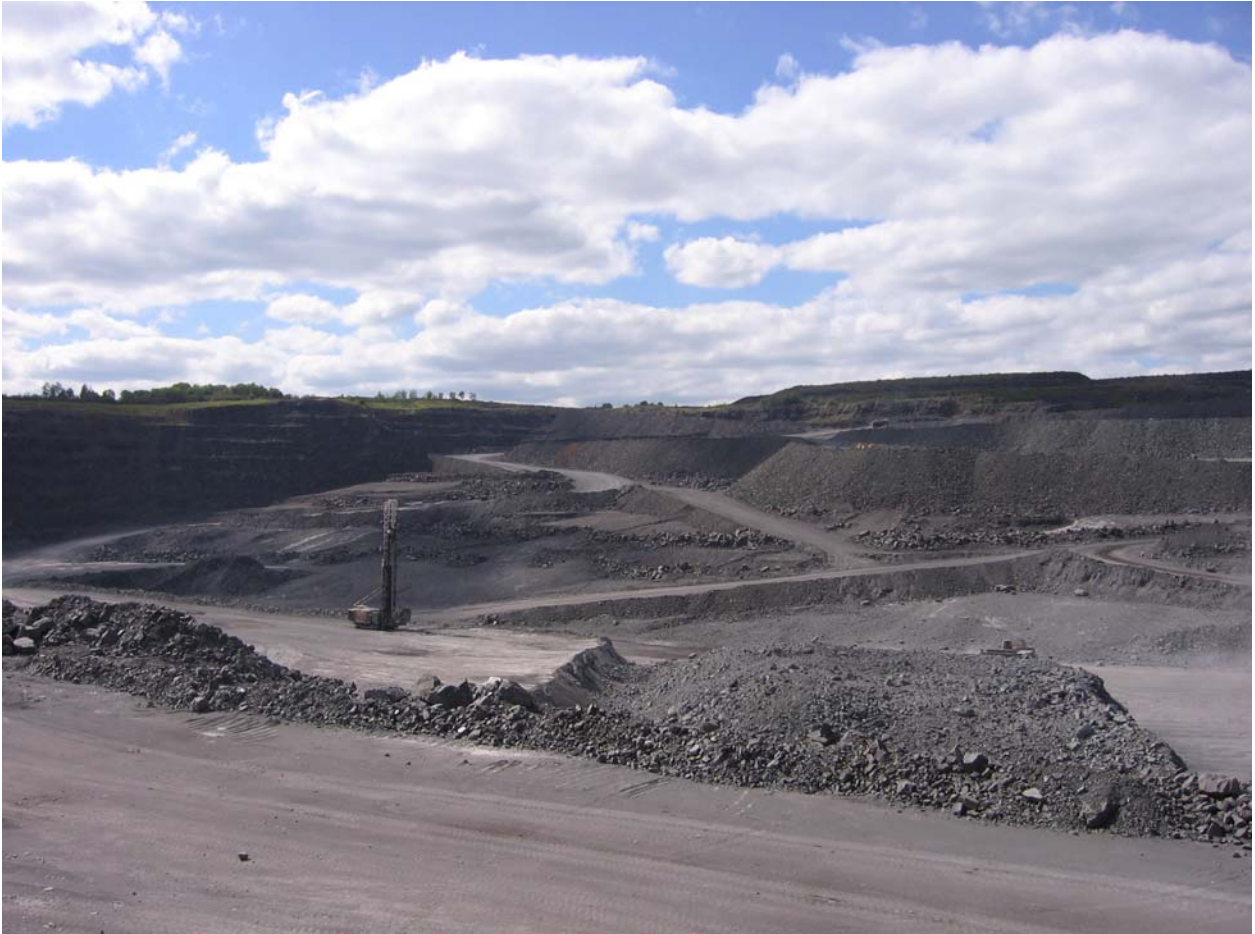
Figure 66. Overall view, looking north, of the Laurentian Mine taken from the uppermost bench of the south wall.
