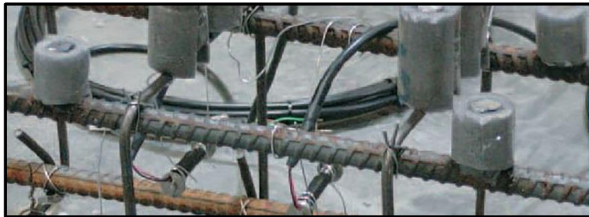
Figure 2-4: Welded, reinforcement stud measurement targets (Smaoui et al. 2007)
