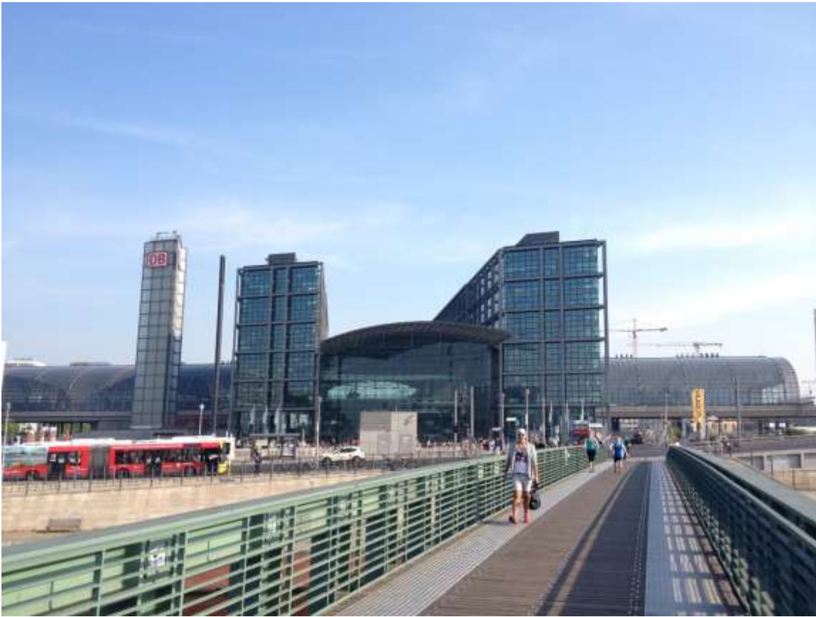
Figure 12: Berlin Hauptbahnhof (Central Train Station)
