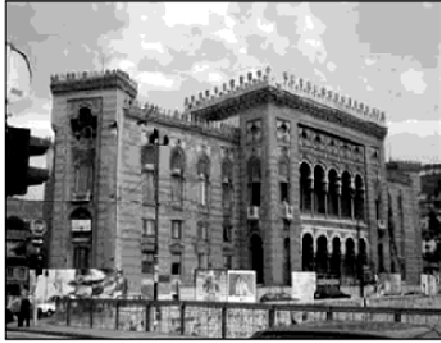
The walls of the National Library (formerly the Town Hall) in Sarajevo, all that is left standing of the library after it was shelled and burned during the war.
